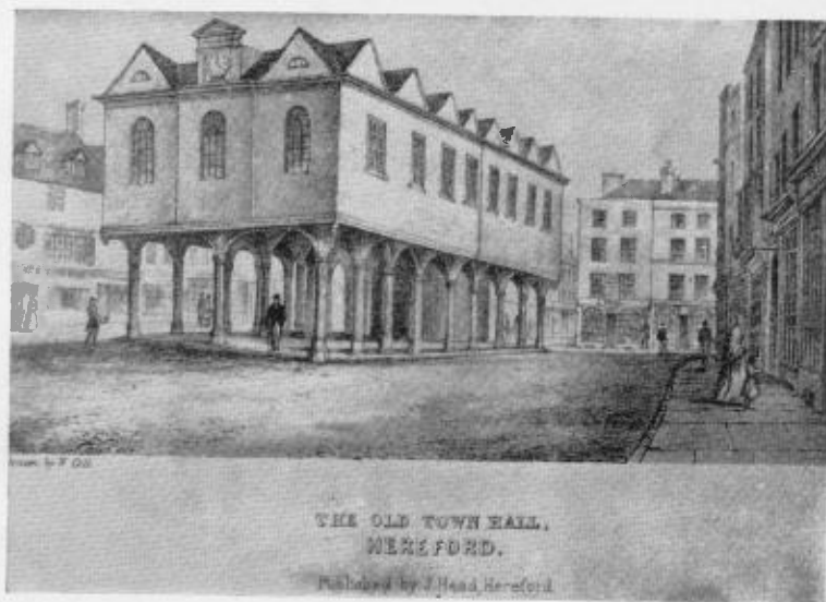
HEREFORD MARKET HALL. EAST END AND NORTH ELEVATION.
