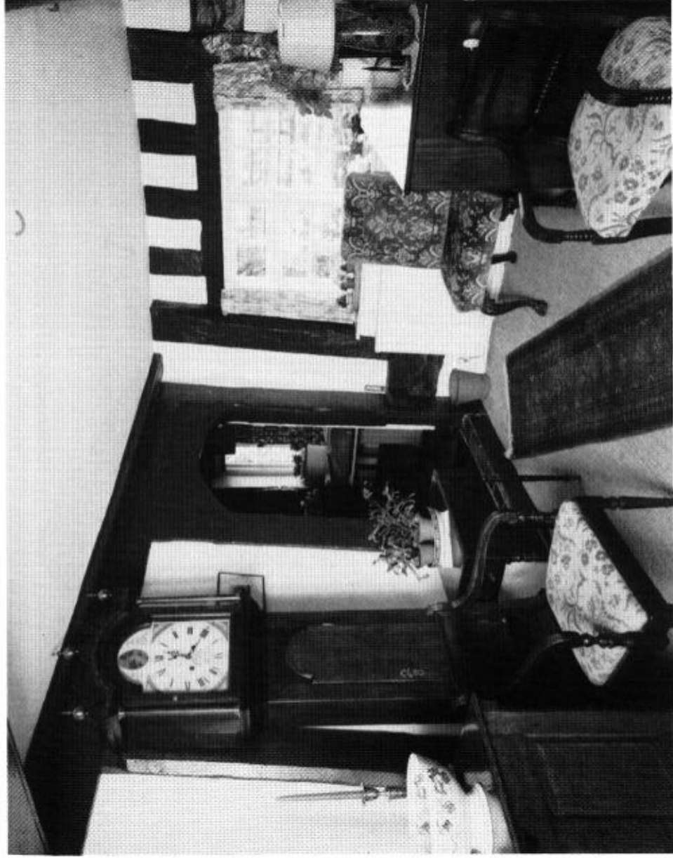
III - The Old House Vowchurch; hall showing doorway to service room, housing (in left jamb) for second door-head, and chamfered stud in partition. (Copyright R.C.H.M.E.).
