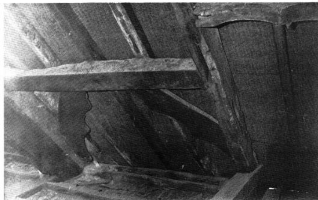
III - Only remaining wind-braces.
