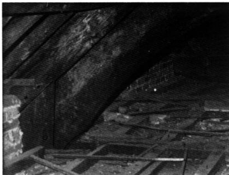
VI - Front post with principal and brace jointed to it.
