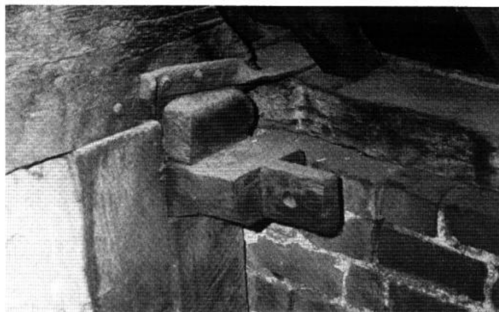
IV - Edge-halved and bridled scarf joint on wall-plate.
