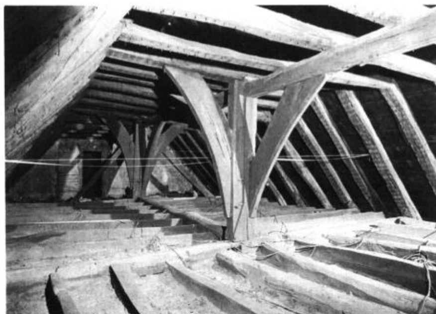
LXXXIV - 20 Church Street - the crown-post roof of c. 1400.
