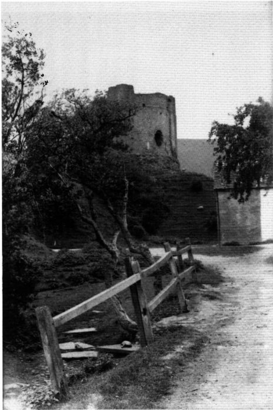
XX - Longtown Castle. Walter de Lacy's great round keep showing the semi-circular projections or lobes. Longtown had three, one being used for a spiral stairway. At Caldicot and Usk there was only one. (Alfred Watkins, F.R.P.S. c.1920)
