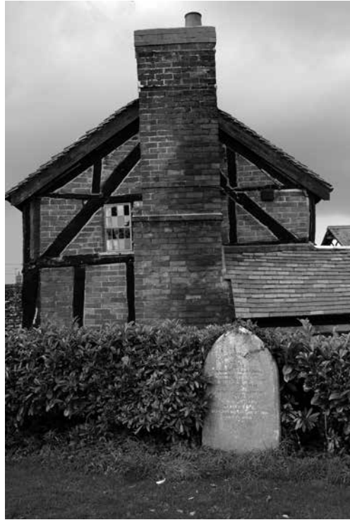
Figure 9. Stepps House, Pembridge. East elevation showing the raised roof.
