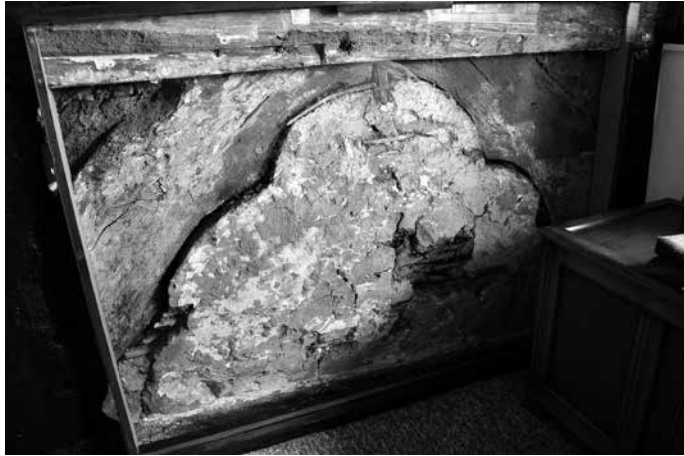
Figure 1. Greenfields, Dilwyn. One of two panels of cusped decoration in the south-east end frame. Above is a rebate for the shutter slide to the adjacent (blocked) window.
