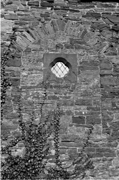
Figure 18. Intramural chamber, showing access from west range.
