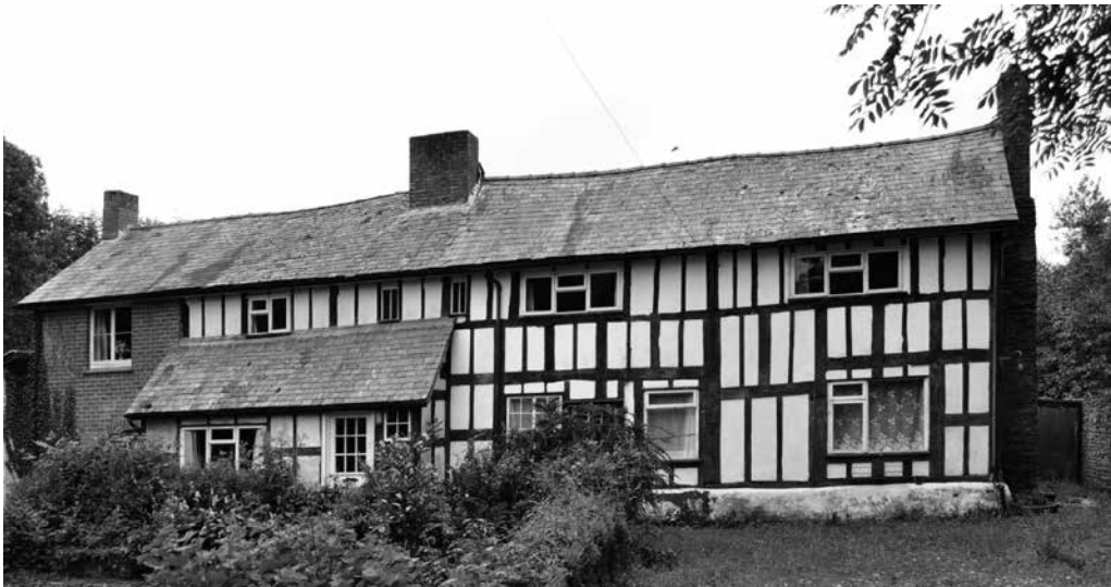
Figure 11. Church House, Titley. The front elevation in 2017. The upper row of windows are a later insertion following the raising of the eaves level. The brick bay and the lean-to are later additions.
