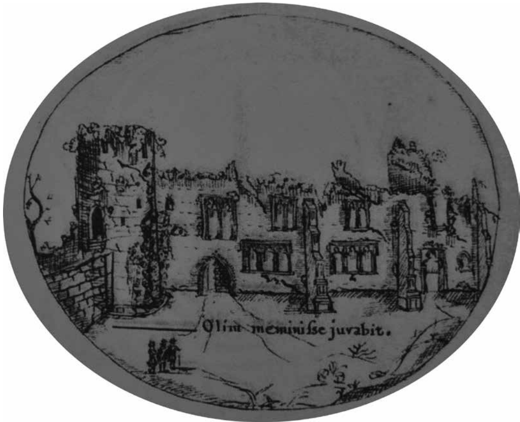
Figure 4. Dingley’s view from the east showing Coningsby’s tower and wall walk
