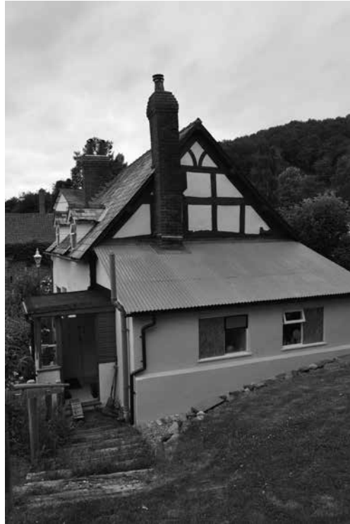
Figure 21. Gayleys, Westhope, Canon Pyon. East elevation tie-beam truss and rebuilt lean-to.
