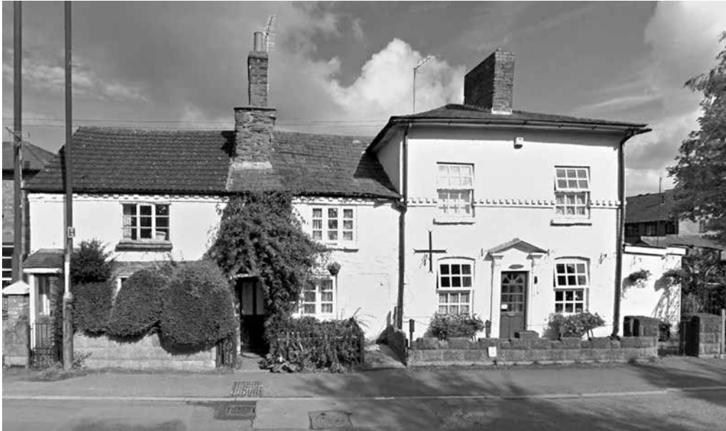
Figure 4. 45-49 Mill St, Leominster.
