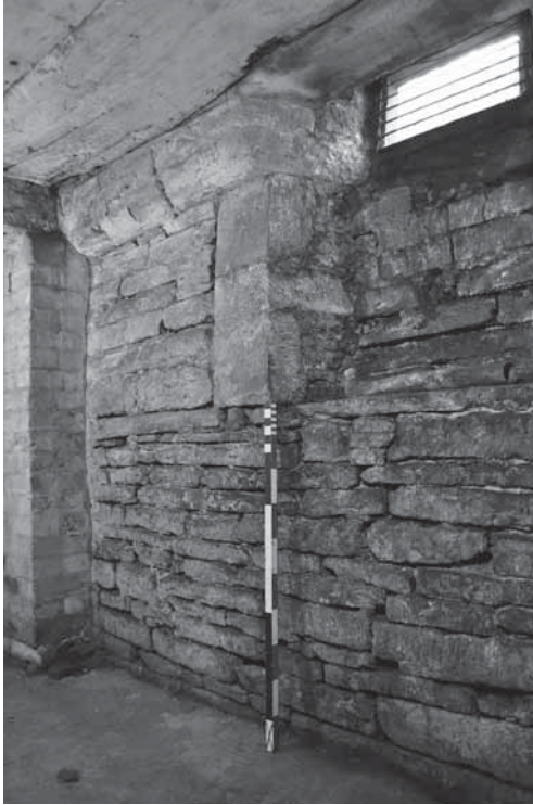
Figure 18. 3 High Street, Weobley. The cellar showing the stonework around one of the two light wells in the north wall.
