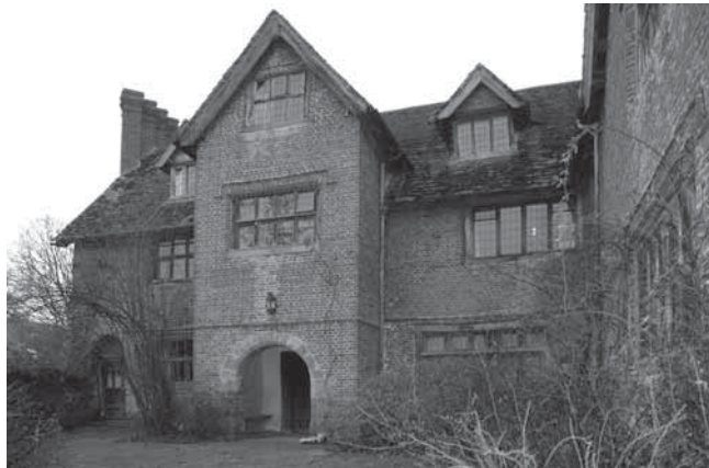
Figure 1. The Rodd, front elevation showing the brick façade and storeyed porch.
