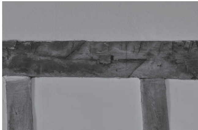
Figure 16. 15 Church Street, Leominster, scarf joint in the top floor tie beam with nailed partition studs below.
