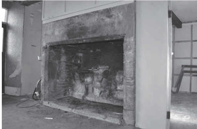
Figure 21. 3 High Street, Weobley. The early fireplace, with stone jambs and lintel.
