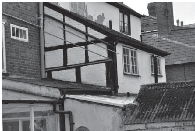
Figure 13. East elevation of the timber framing at the back of 11 Church Street, marked in grey to indicate the earlier roof level.
