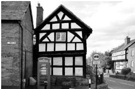
Figure 14. The jettied south end of the range with 17th-century framing inserted below the jetty
