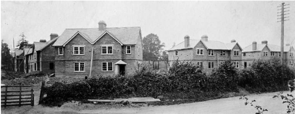
Figure 9. Houses under construction on Ross Road
