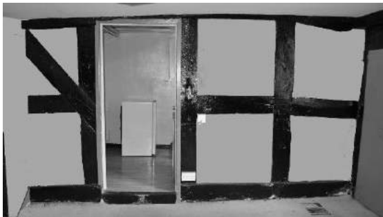
Figure 12. Bay 7 looking north at the inserted 17th-century crossframe on the ground floor
