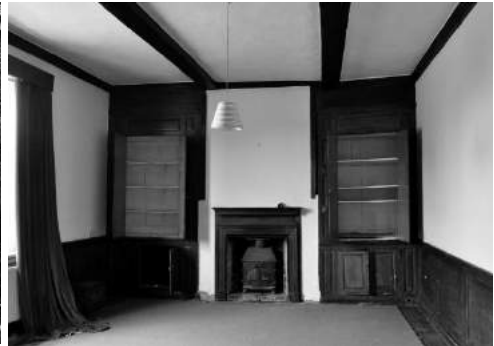
Figure 26. Room 4, looking north-east at the inserted chimneystack and cupboards
