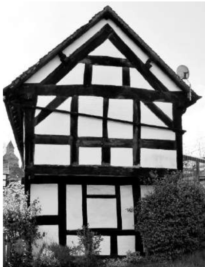
Figure 8. The jettied north elevation of the range showing the blocked window openings
