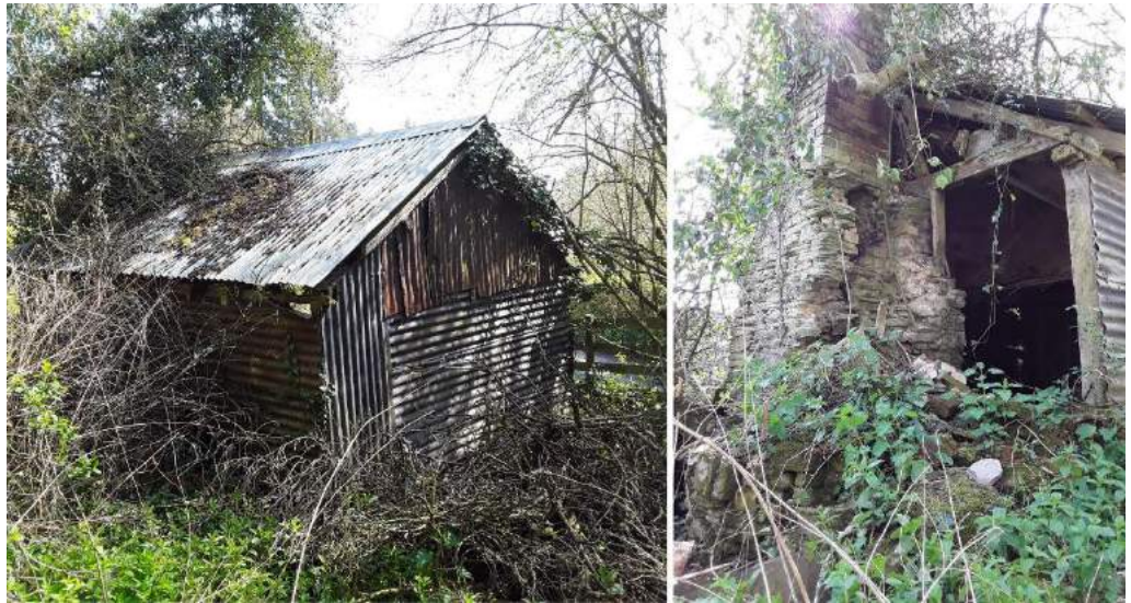
Plate 5.2. Two views of the possible toll house at The Old Shop, Lingen
