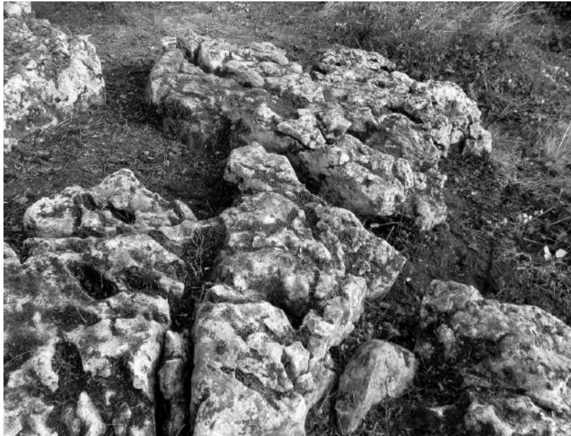
Figure 6. Eroded surface of limestone pavement which has been exposed for many years
