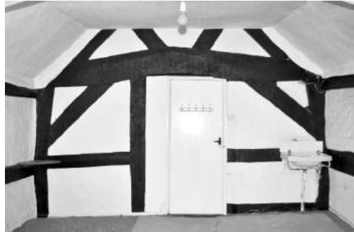
Figure 11. Bay 2 looking south to truss T3 with its vee-struts and massive cambered tiebeam
