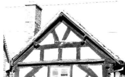
Figure 15. The south end gable showing the clasped purlins in truss T8
