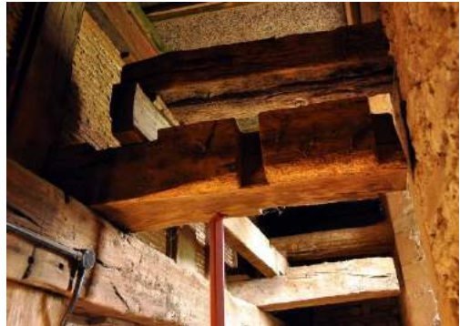
Plate 10.4 (above) Behind the south frame showing that the two north-south beams don't engage with the wall of the tower although they achieve an indirect link through an arrangement of beams above
