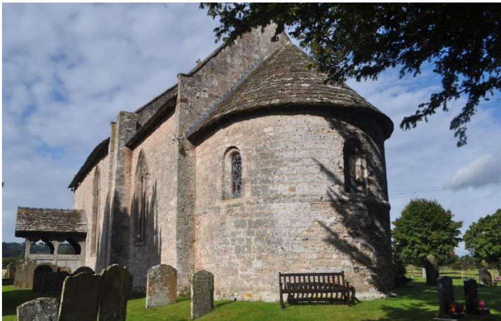
Plate 6.2. St Michael's from the south-east – a two-celled church with an apse. The masonry carefully restored under the supervision of George Gilbert Scott junior in 1870 (D. Whitehead)
