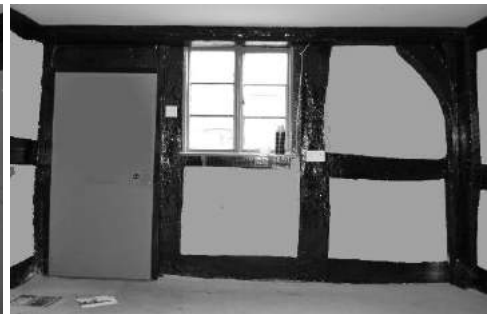
Figure 13. Bay 7 looking east showing one half of a curved doorhead related to the former use of the cross-wing in association with a hall range
