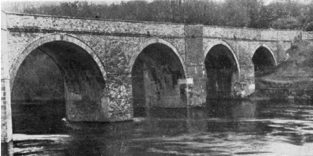
Figure 4. Bredwardine Bridge after restoration: a photograph published in the volume of the Transactions for 1924-6 (Plate 40.)
