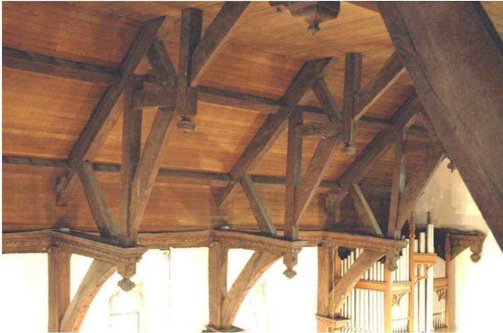
Plate 10.1 (above). The lower two hammer beams of the unorthodox triple hammer-beam roof in Brampton Bryan church
