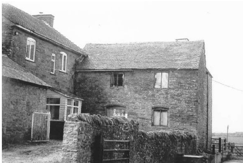
Figure 2. Copley Farm, Cradley, cider mill attached to house; rear hop kiln erected later
