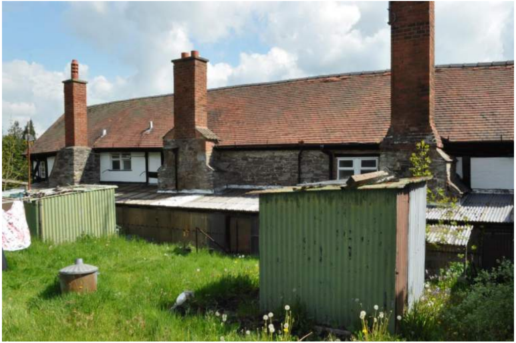
Plate 10.6. The rear elevation of the range showing the three large chimney stacks. Note the higher ground level that had to be cut back to create a level platform for the building
