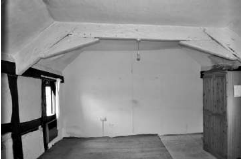
Figure 10. Bay 2 looking north showing the intermediate roof truss between bays 1 and 2
