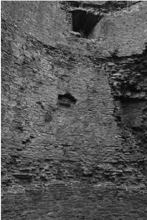
Figure 9. Longtown Castle showing floor joist support and entrance to garderobe.
