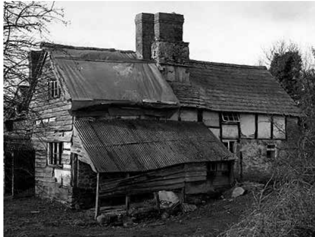
Figure 4. Bruton Farmhouse. East elevation showing the building in derelict condition, c.2000, prior to repair.
