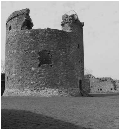
Figure 5. Dundrum Keep from south, showing first-floor entrance and wall walk.
