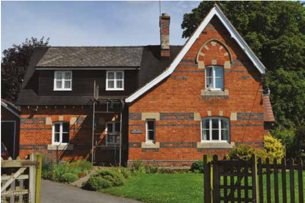
Plate 4.1. Westside School (1863): classroom left (heightened), master's house right.
