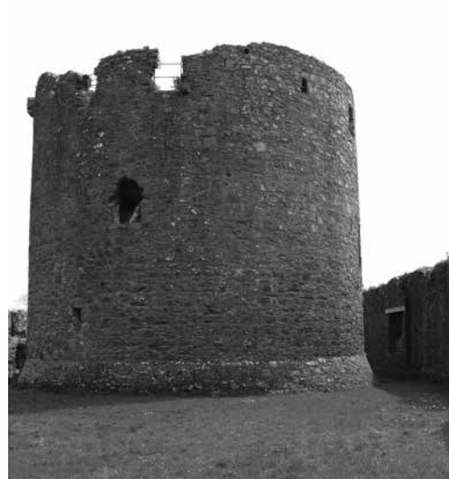
Figure 6. Dundrum Keep from north, showing battered base and, right, latrine in curtain wall.
