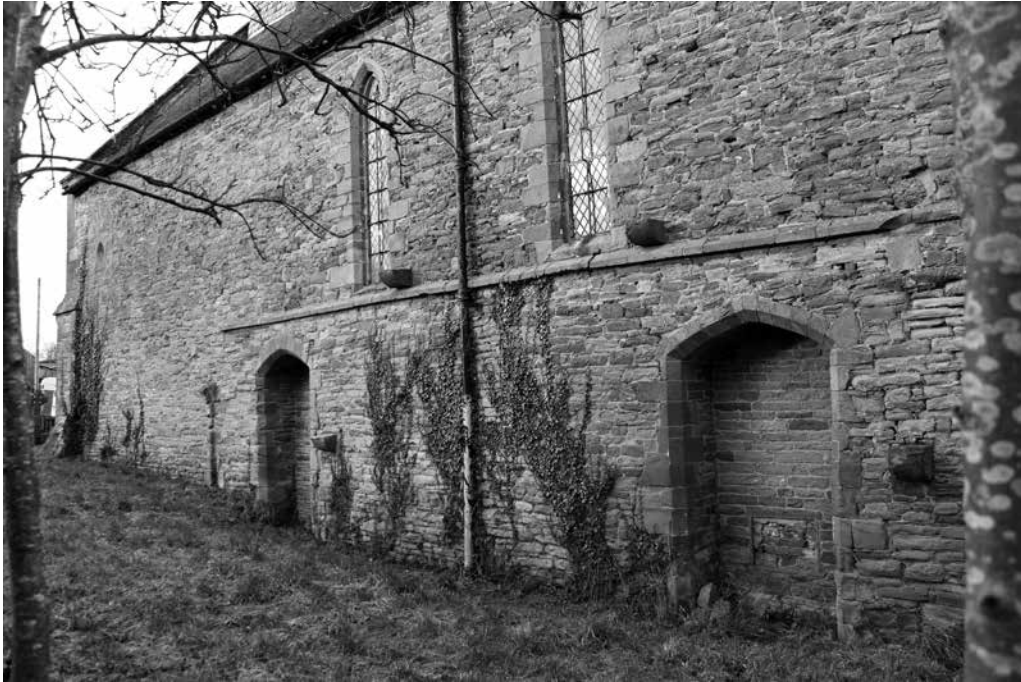
Figure 3. Aconbury Church. South face showing cloister string course, nuns' entry left, priests' entry right.
