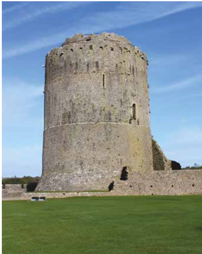
Plate 3.3 Pembroke Castle. William Marshal's 75-ft high circular keep showing remains of domical roof and heavy battery at base.
