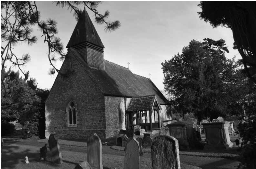
Figure 6. Putley Church (1875). Blashill renewed the belfry and strengthened the west wall for support. He added the west window. The timber porch shown by Wathen was also restored but was replaced in c.1940
