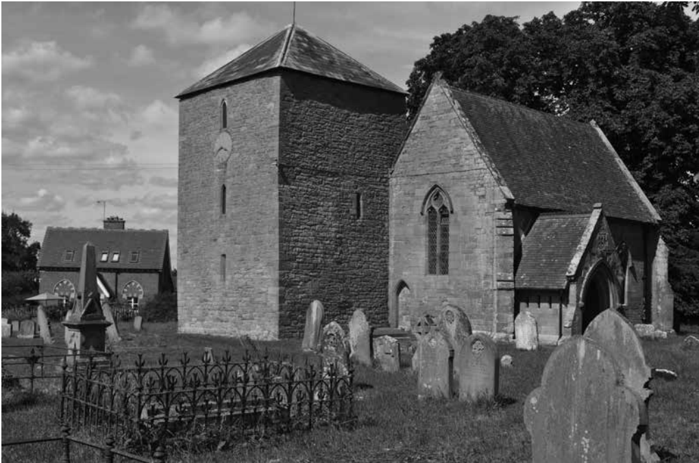
Figure 3. Westhide Church (1866-7). View of the south-side where Blashill consolidated the masonry, opened-up the easternmost window and designed a new porch. The tower was restored in c.1870.
