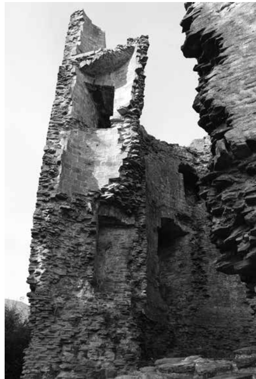
Figure 11. Longtown Castle: remnants of southern buttress showing spiral staircase and opening into dog-legged passageway on 2nd floor.
