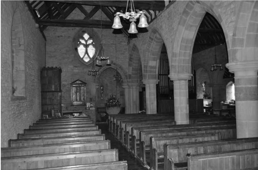
Figure 4. Stottesdon Church (1867-8). The new baptistery designed by Blashill to show-off the font. A new ox-eye window was provided to illuminate the scene.
