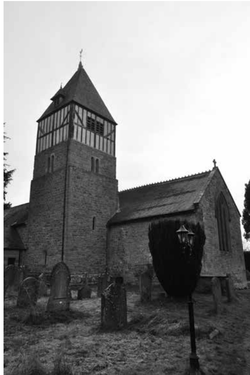
Figure 10. Hampton Bishop (1878-9). The north side of the church, showing the tower, restored by both Kempson (1866) and Blashill (1878). The third storey with its 'Norman' openings was designed by Blashill. He also cleaned and restored the stonework below.
