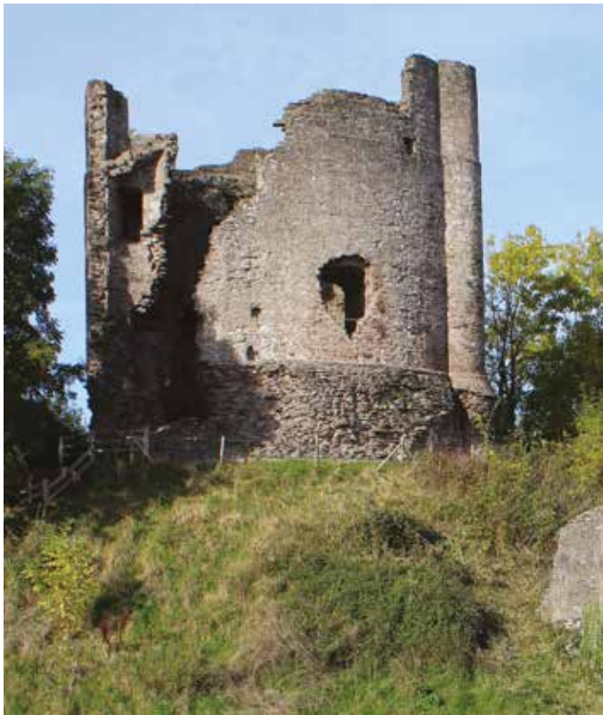
Plate 3.6. Longtown Castle on its motte, viewed from the south, showing two of the three semi-circular buttresses.
