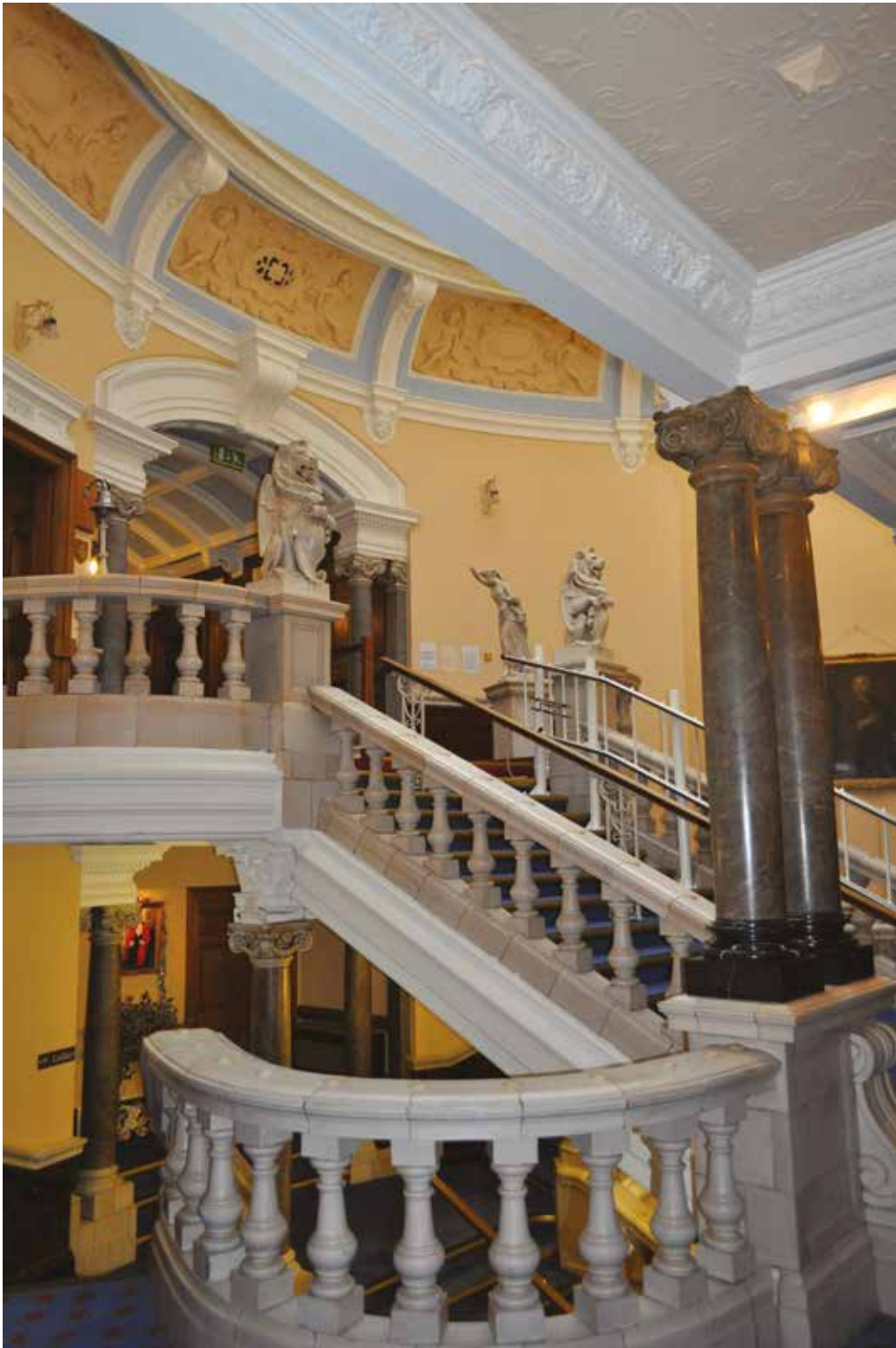
Plate 4.5. Hereford Town Hall, The 'Imperial' staircase: Doulton's best terracotta, York stone, black marble columns and top-lit with Art Nouveau stained glass—posh qualities that would elevate any bride's wedding day.
