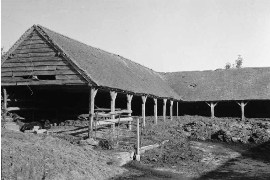
Figure 12. Shelter shed, Hill End Court, Castlemorton (W).
