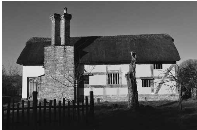
Figure 6. Hacton Cruck cottage. East elevation of the refurbished building. The middle bay is the hall and on the right is the solar bay. The left-hand bay and chimneystack are modern additions.
