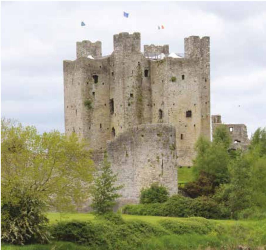
Plate 3.1. Trim Castle, built by Walter's father, 1174-86. Fundamentally a square keep to which four rectangular towers were subsequently attached. These are shown projecting above the keep.
