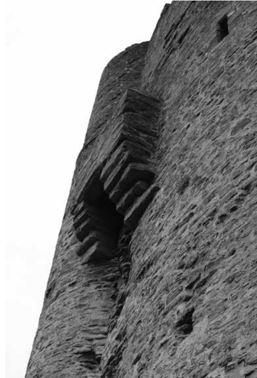
Figure 13. Longtown Castle, showing projecting rectilinear corbelled-out garderobe.
