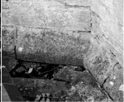
Figure 6. Return in the plinth moulding underpinning the joint between the east wall of the south transept and the rood loft stair tower
