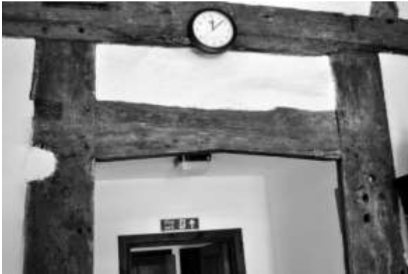
Figure 2. The Ale House, Colwall. Following the addition of the later, east bay the original doorway is now internal
