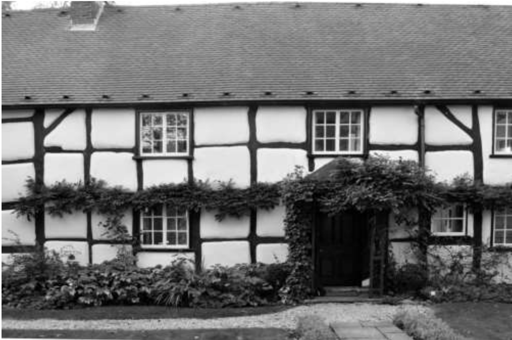
Figure 13. Winterslow, Church Road, Colwall. The two middle bays forming the primary structure
