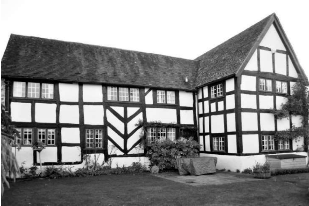
Figure 10. Upper House, Evendine Lane, Colwall. West elevation of the main range and crosswing
