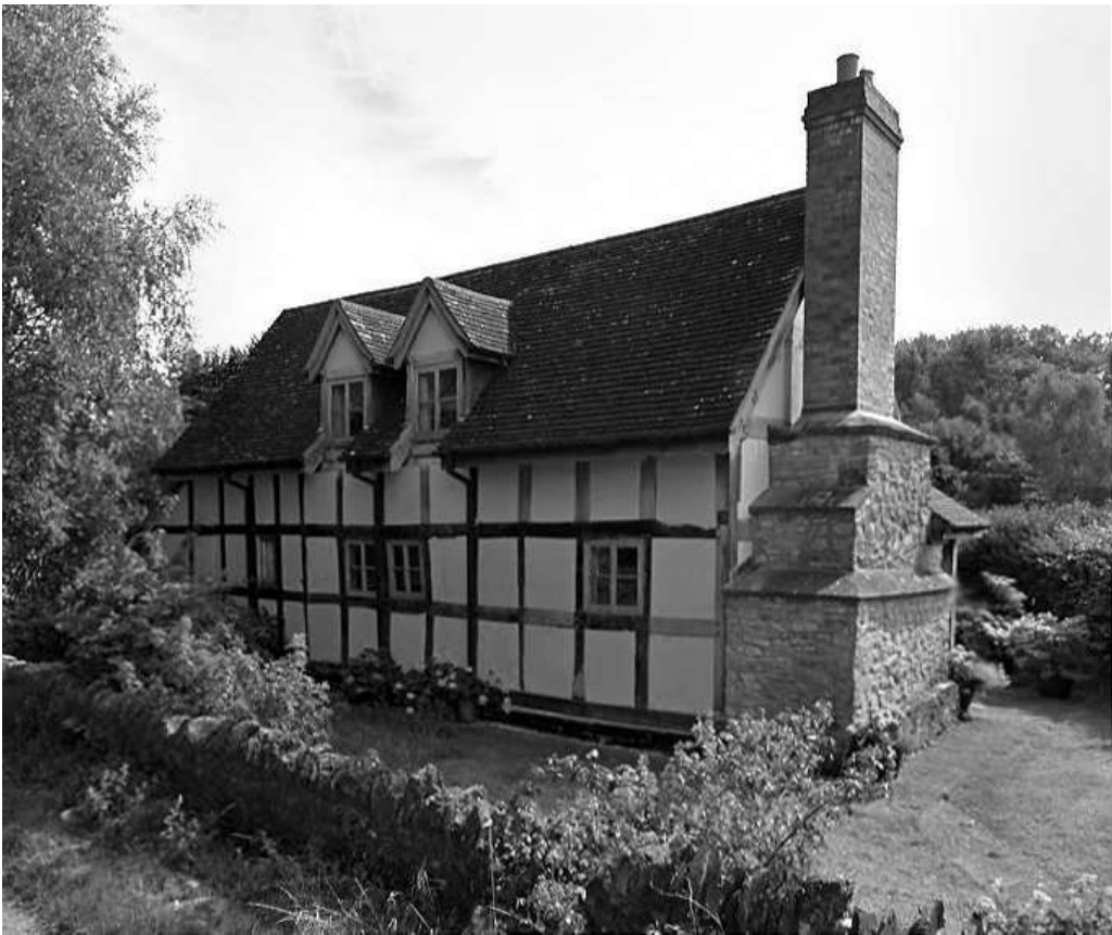
Figure 8. Peaty Cottage, Church Road, Colwall, with its massive external chimney stack
