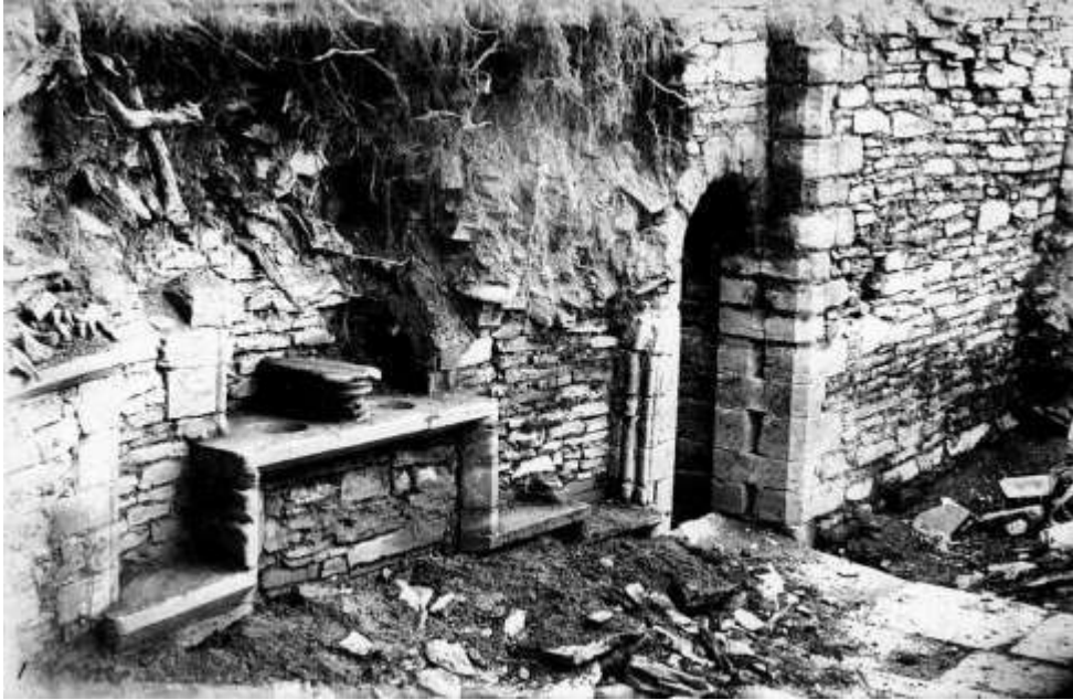
Figure 17. Credence, piscina, sedilia and door to south chapel, showing southern reveal. Photo A. Watkins, TWNFC (1904), Fig. 32
