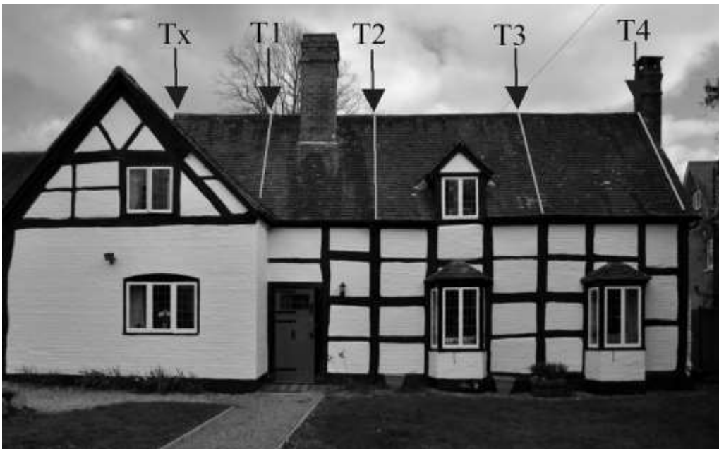
Figure 9. Stone Holt, Walwyn Road, Colwall, showing the positions of the roof trusses
