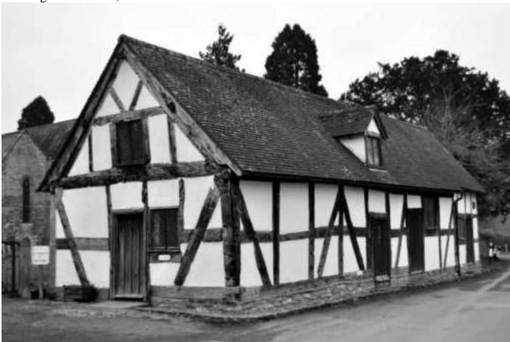
Figure 1. The Ale House, Colwall, was constructed as a two-storey jettied building. The later bay at the far end was added after the jettied upper storey had been removed. The present gable-end doorway is a later insertion.
