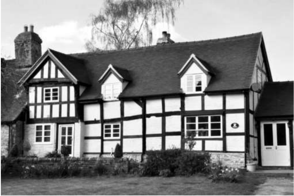
Figure 19. The Forge, Lingen, to the east of Mortimer Cottage
