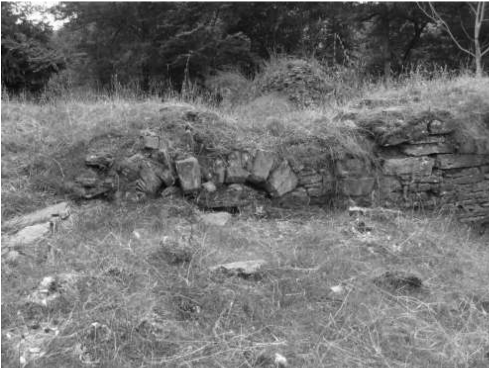
Figure 33. South chapel showing head of piscina and southern reveal
