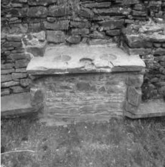
Figure 37. Piscina after conservation work in 2014
