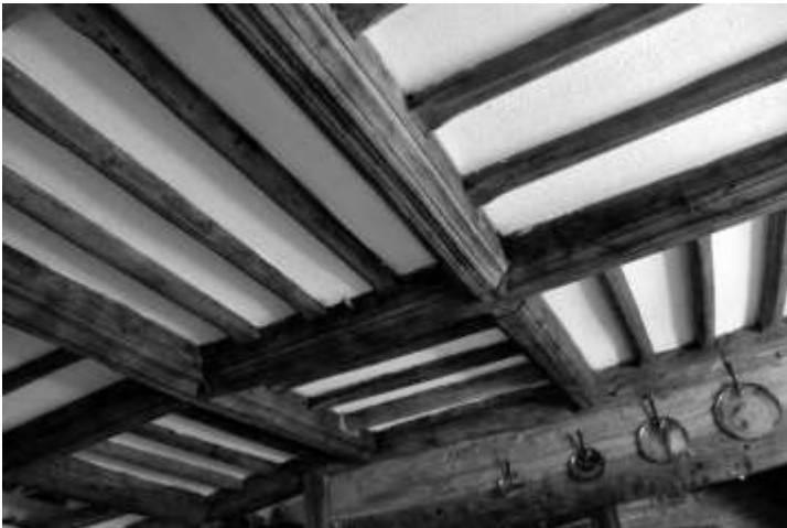
Figure 17. Mortimer Cottage, the moulded beams
