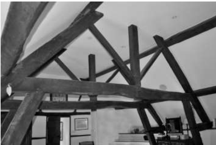
Figure 12. Roof trusses in the former coach house
