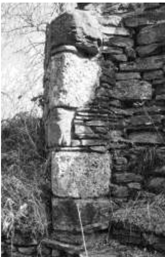
Figure 15. South apse window, tufa strengthening of southern side
