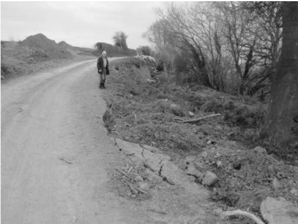
Figure 1. The landslide at Shortwood Farm. The land below the drive dropped
