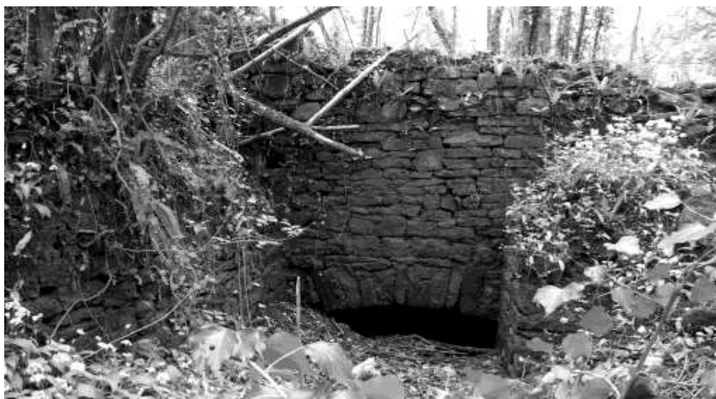
Figure 9. The exit of the culvert which carried water from the forge pool under the forge. It is possible that there was a wheel-pit here for the wheel at the downstream end of the culvert. (Photo: R. Lowe)
