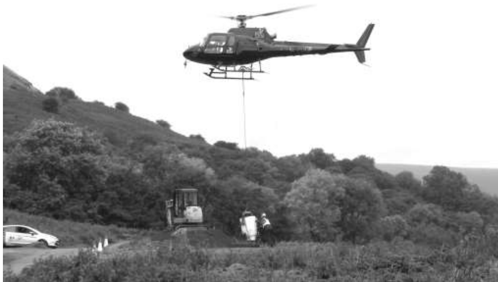
Figure 4. Helicopter at Black Darren picnic site working to repair the Offa's Dyke Path and to conserve peat deposits
