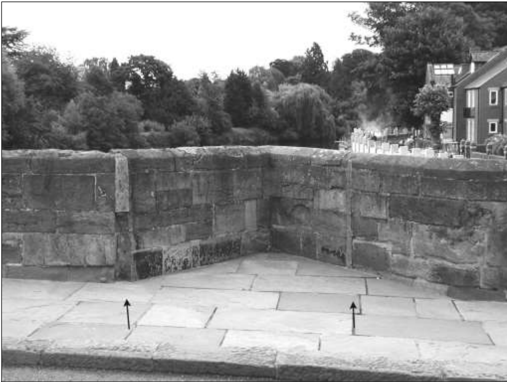
Figure 1. The two grooves cut into the sides of the refuge
