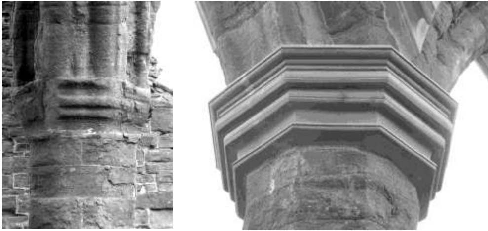
Figure 5 (left). The central capital on the Solar Arch at Goodrich castle showing the extent of decay Figure 6. (right). The replaced capital
