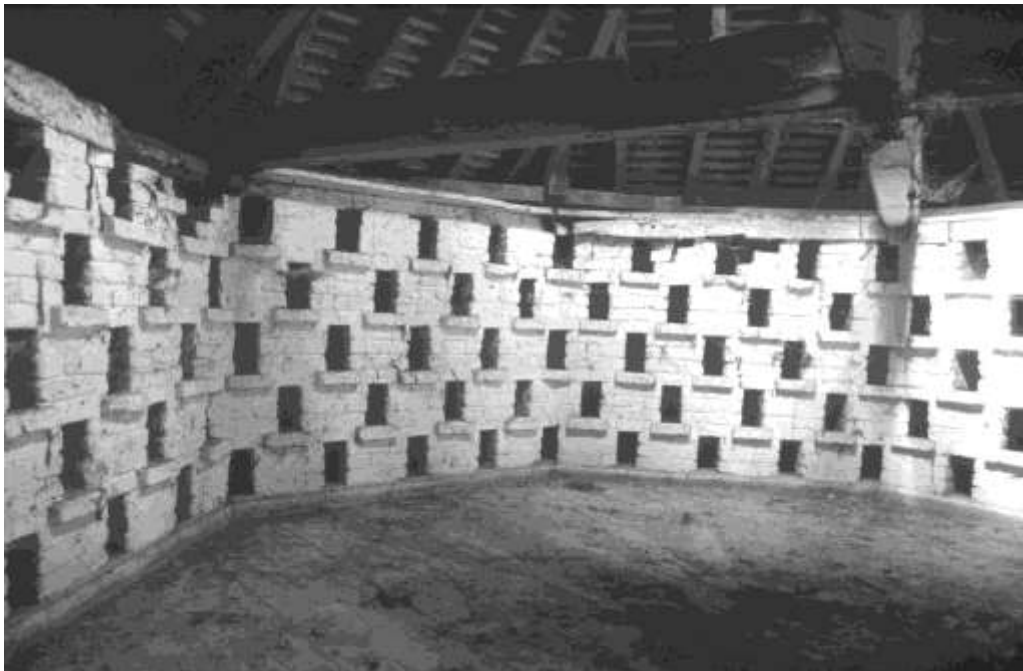
Figure 5. The five upper tiers of nest-holes and the halved tie-beams which supported the upper bearing of the revolving ladder (John McCann)
