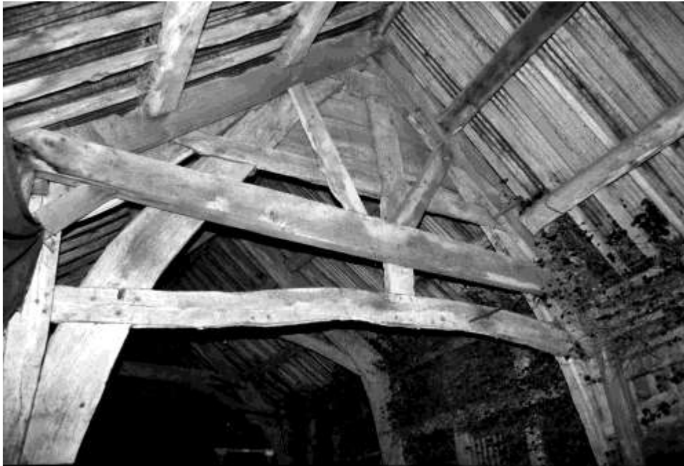
Figure 5. Barn at Weston Court, Pembridge in 2003. Part of the gable framing of the cruck barn has been removed to allow access to a late 17th/early 18th century addition, at one time used as a cowhouse with loft above. During the 19th century two further additions were made, one a stable. The extensive range of mainly timber framed barns and shelter sheds at Weston Court is now being converted to residential use
