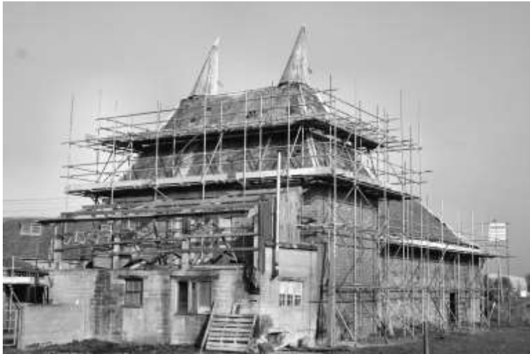
Figure 9. Brookhouse Farm, Moreton on Lugg in 2005. The twin hop kilns of brick, attached to a stone cider house, were present in 1904 but the greenstage is later. Now in residential use
