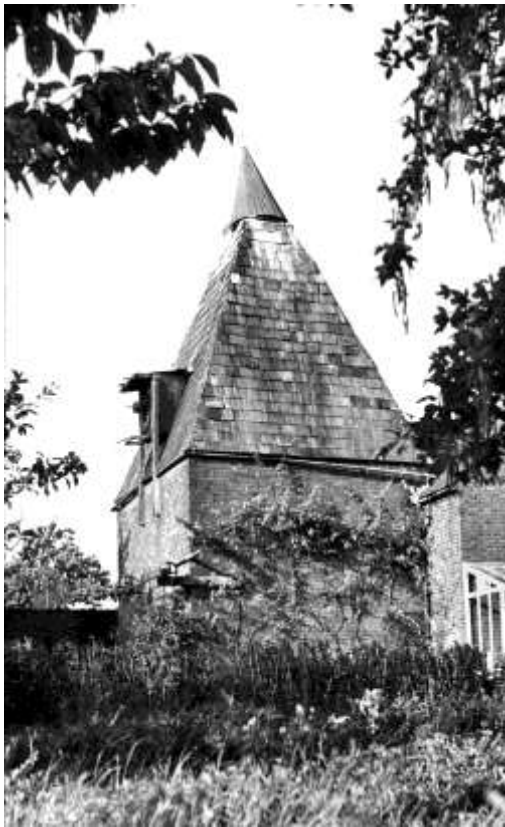
Figure 11. Hop kiln at Eastwood Farm, Tarrington in 1973. The inserted top fan was belt-driven by a stationary engine. Now in residential use
