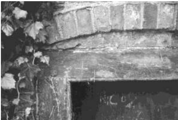
Figure 3. The brick arch and pegged oak door-frame (Frank Pexton).
