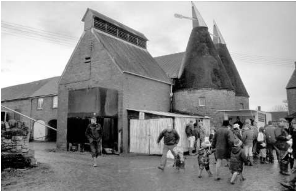
Figure 8. Brook Farm, Little Marcle in 2002. The round hop kilns are stone, with brick dressings, and the conical roofs are of brickwork, weatherproofed with pitch. The rectangular kiln with louvered ridge was ‘modern’ in 1916; a building was mapped on this site in 1904. Now in residential use
