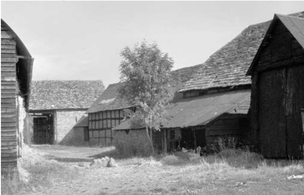
Figure 1. Farm buildings at Black Hall, Kings Pyon in 1973, now demolished. A farmstead of wide date range, using a variety of building materials. Timbers from the 4-bay cruck barn (extreme right) had a felling date range of 1440-1476 ( Vernacular Architecture , 31, p.115.). The lean-to on the left of the porch housed an engine for driving barn machinery. The Dutch barn (extreme left) is c.1912
