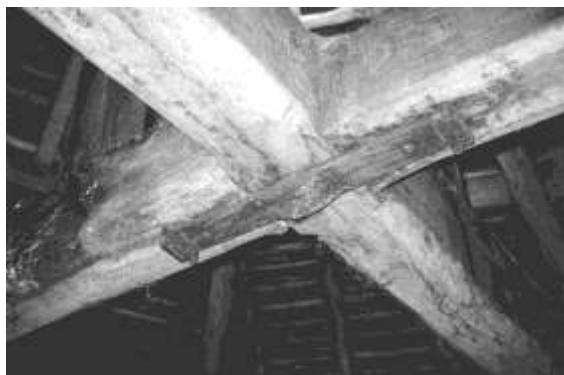
Figure 8. The upper bearing of the revolving ladder
