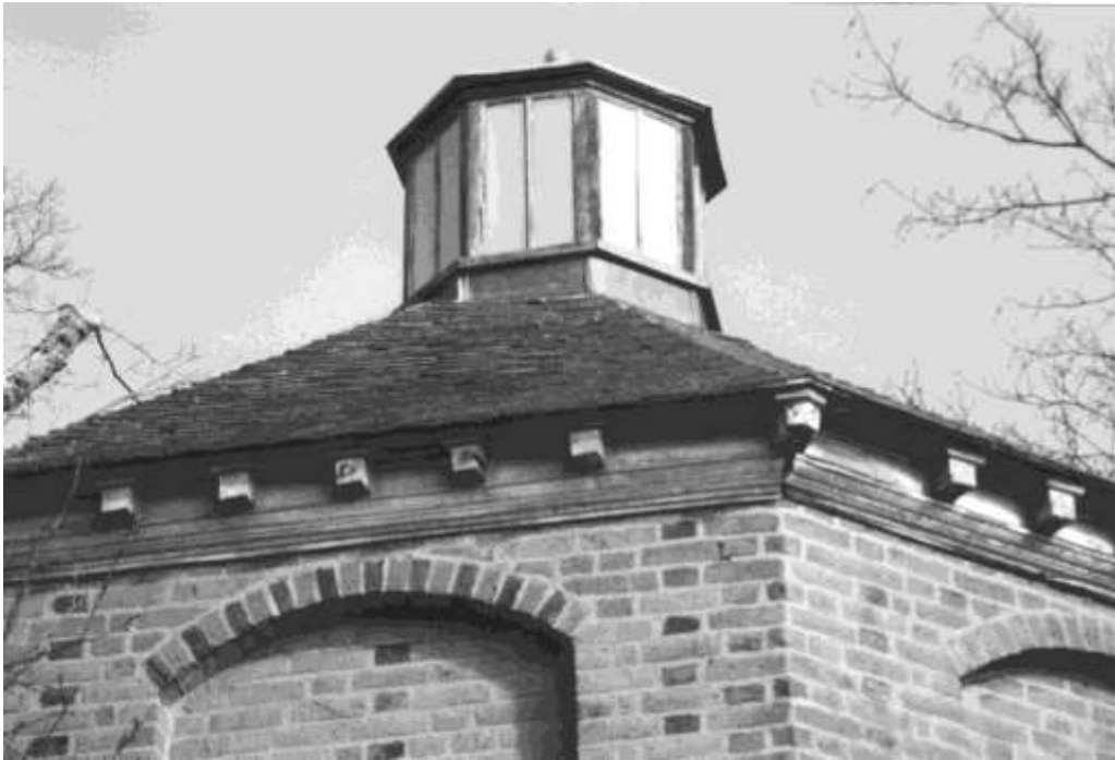
Figure 2. The roof and lantern, converted from the original louver. Note the decorative use of blue headers in the brickwork, the moulded cornice and the wooden dentils (Frank Pexton)
