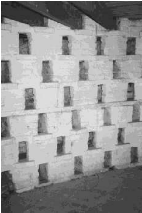
Figure 6. Nest-holes in the present middle storey, showing the bonding course which forms a continuous alighting ledge (Frank Pexton)
