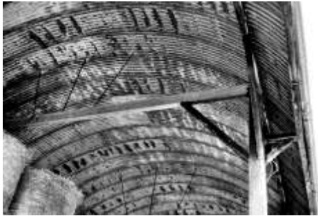
Figure 13. The most common type of Herefordshire Dutch barn construction; the extended eaves date it after 1912
