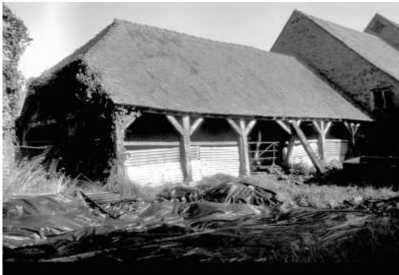
Figure 7. A possible sheepcot in the Leadon valley in 1985. There is a loading door in the gable of the loft. The broad ceiling joists which carry the wattle floor of the loft are laid flat
