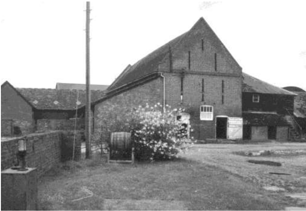
Figure 3. Monksbury Court, Yarkhill in 2000. The brick barn, built between 1778 and 1790, incorporated a stable with loft above. The far gable has raised brick detailing, and the tie beams are re-used cruck blades. Now in residential use
