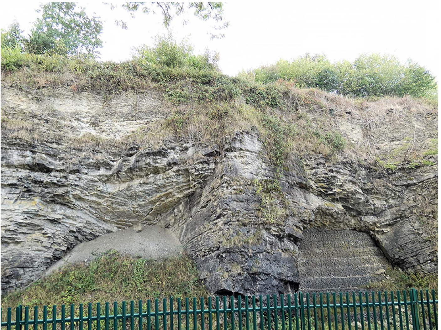
Figure 4. Showing three large pillars and two tunnel entrances with the right hand tunnel blocked with stone cases with a small opening near the top to let the bats come and go in this limestone cavern.
