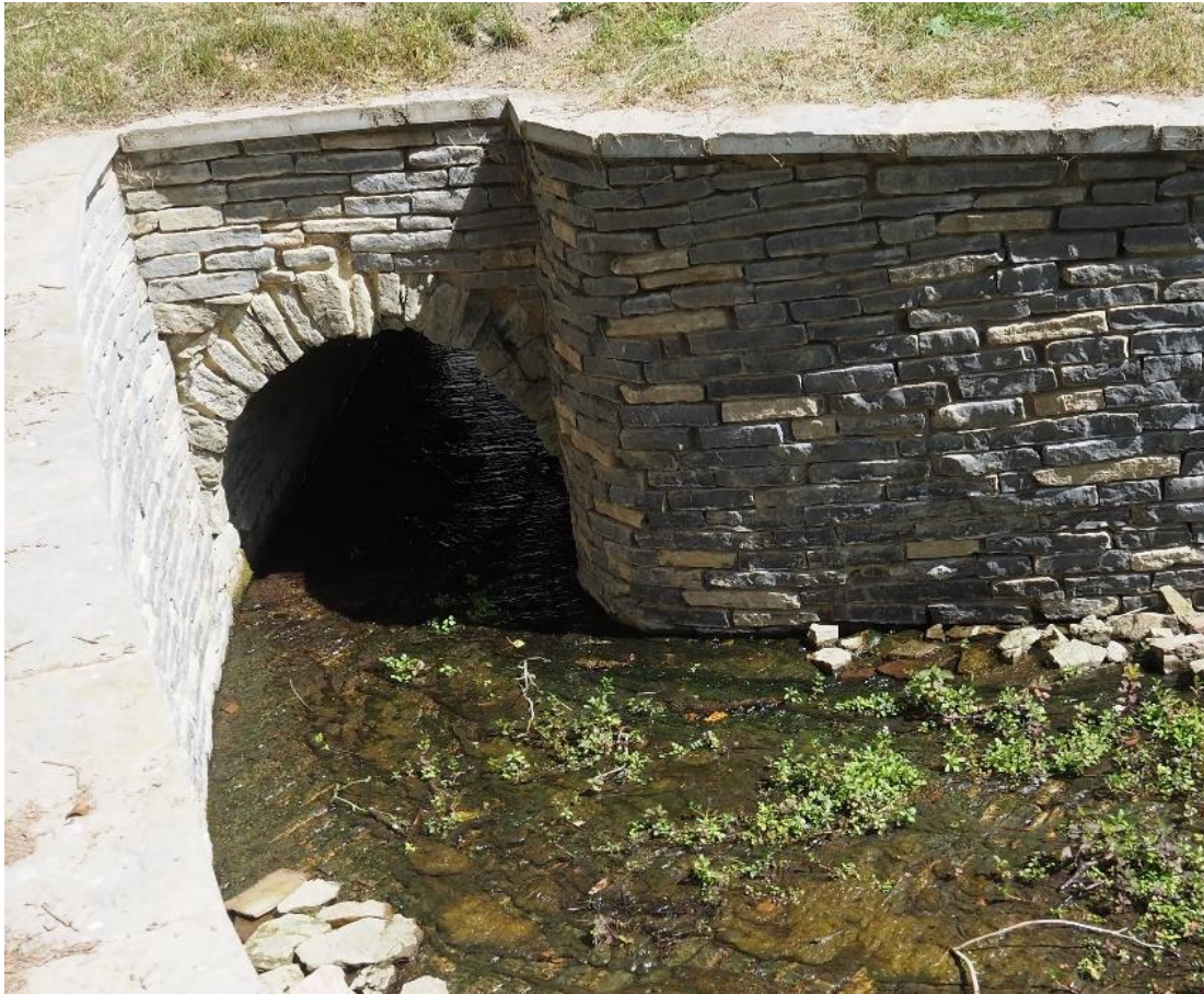
Figure 5. Fishpool Valley, tunnel to allow crayfish to move between the pools
