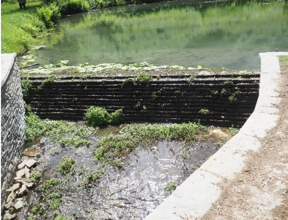
Figure 4. Fishpool Valley, cascade built into a dam
