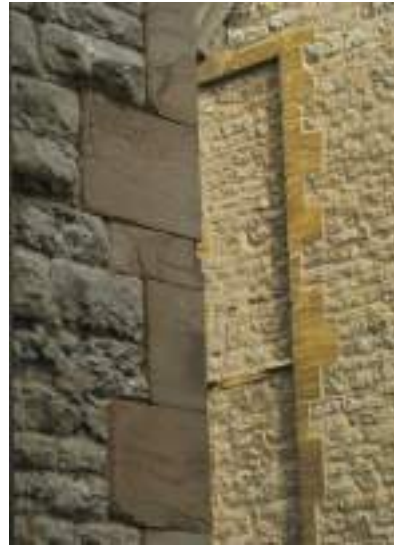
Contrasting colours of the sandstone quoins in the old library and the almshouses in Ledbury.
