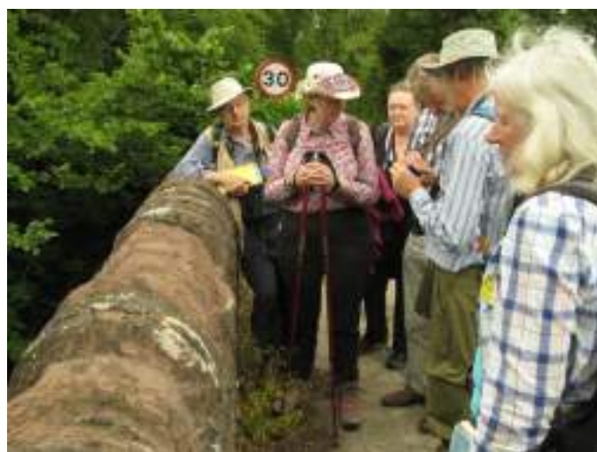
The party discusses the stone erosion at the Goodrich road bridge
