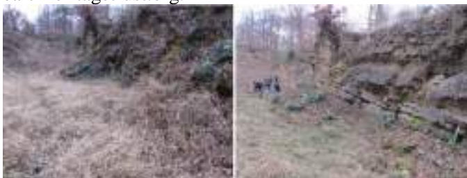
Rudge End Quarry. Left: Main face before clearance. Right: The cleared rock face and stinking hellebore
