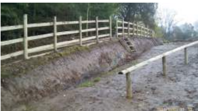
Fig. 1 : New fencing at the site
