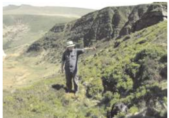
Duncan stands on a collapsing block at the top of the landslide. Behind are the southern cliffs of the Cwm and, to the left, the peaks of the Brecon Beacons.
