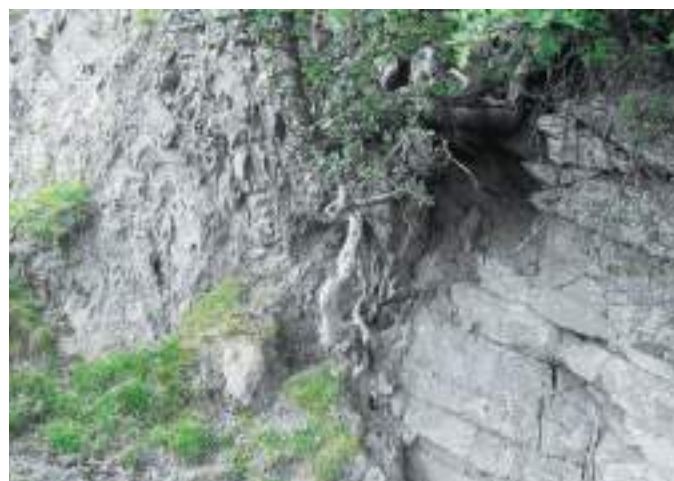
Fig 7 : Fault zone with sheared rock associated with the Church Stretton Fault Complex
