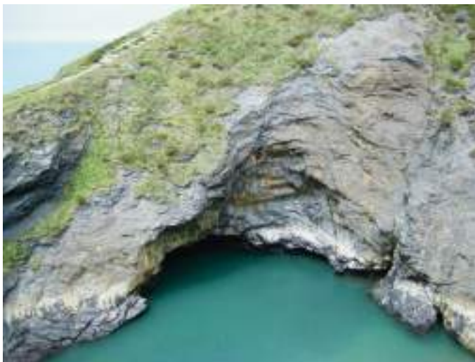
Fig. 4 : Collapsed sea-cave ('The Witch's Cauldron') near Ceibwr Bay
