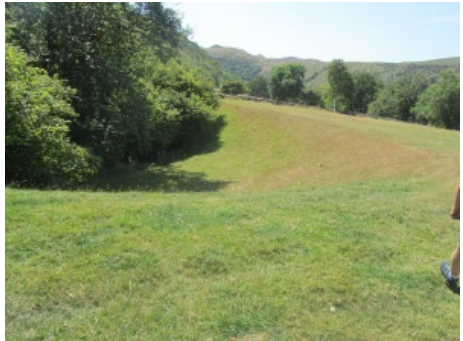
Sinkhole at Pwllcoediog
