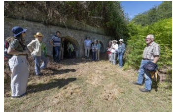
Restored lime kilns, Kentchurch
