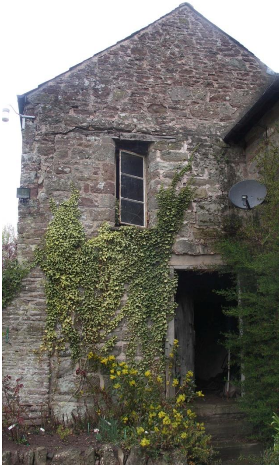
Figure 20. East face of 'barn'
