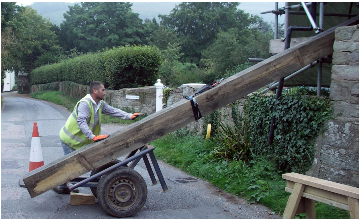
Figure 17. New sole plate being manoeuvred into position
