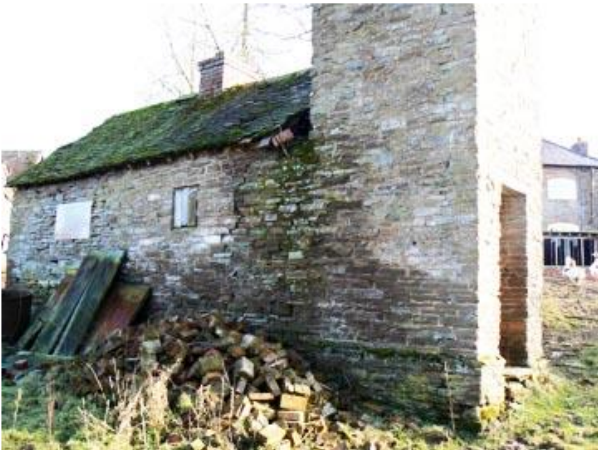
Figure 26. Bell tower showing plinth
