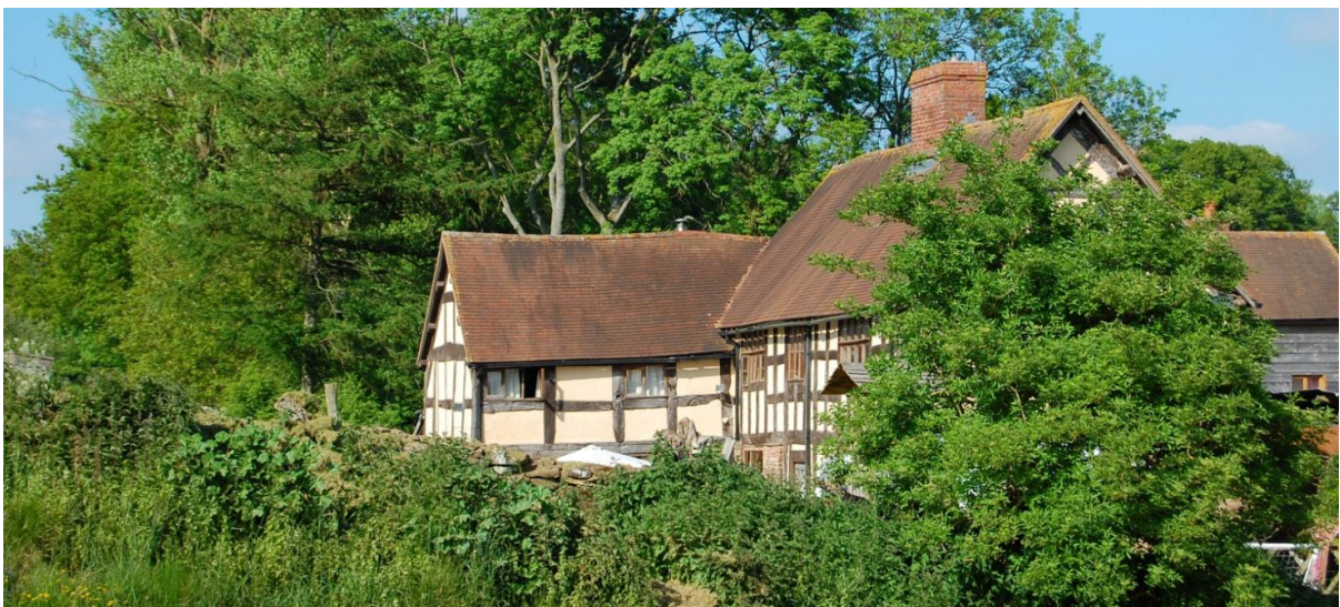
Figure 9. Lower Buckland showing cross-wing with older, larger timber-framing than the main house
