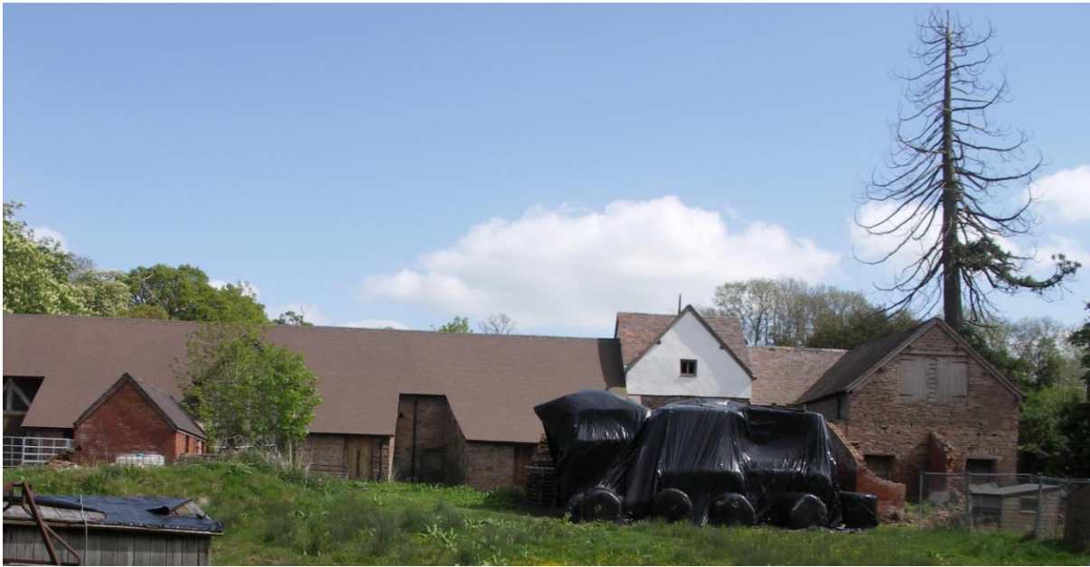
Figure 56. The rear of the farm building range.
