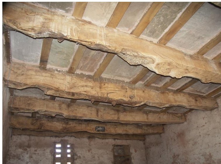
Figure 15. The roughly-cut joists in the cart shed under the dovecote.
