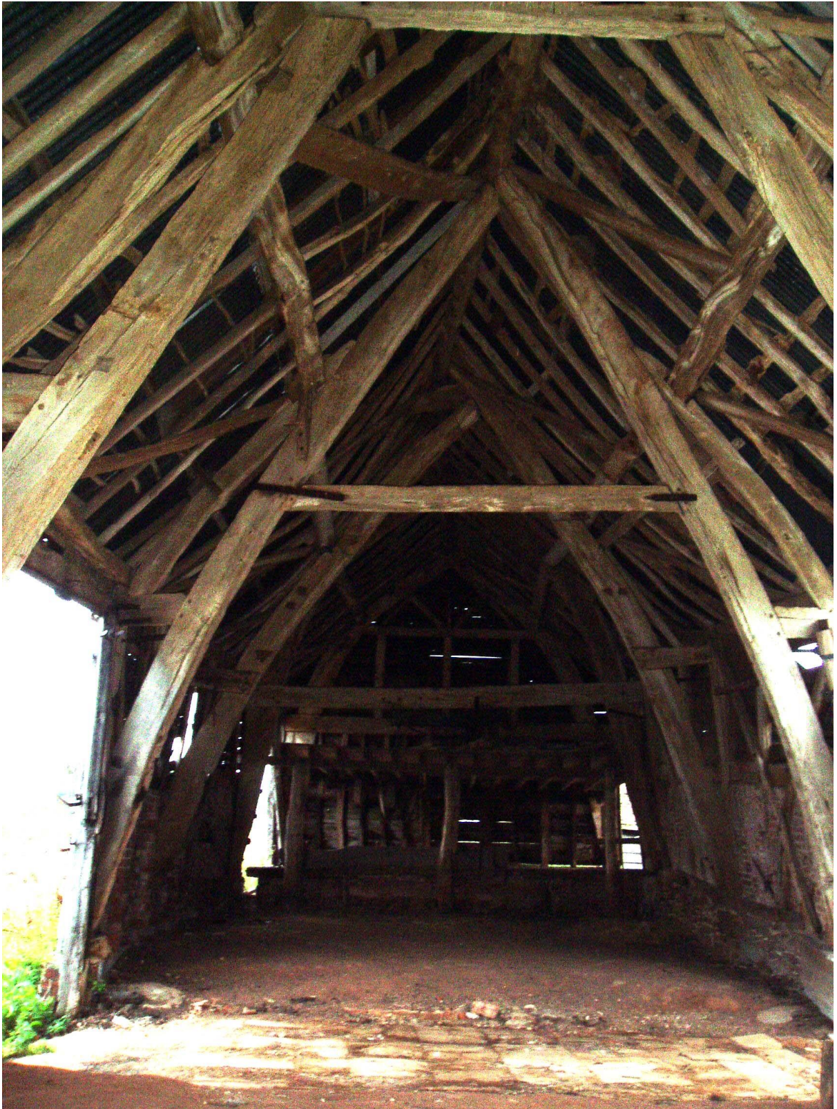
Figure 6. The interior of the barn after clearance but before work started
