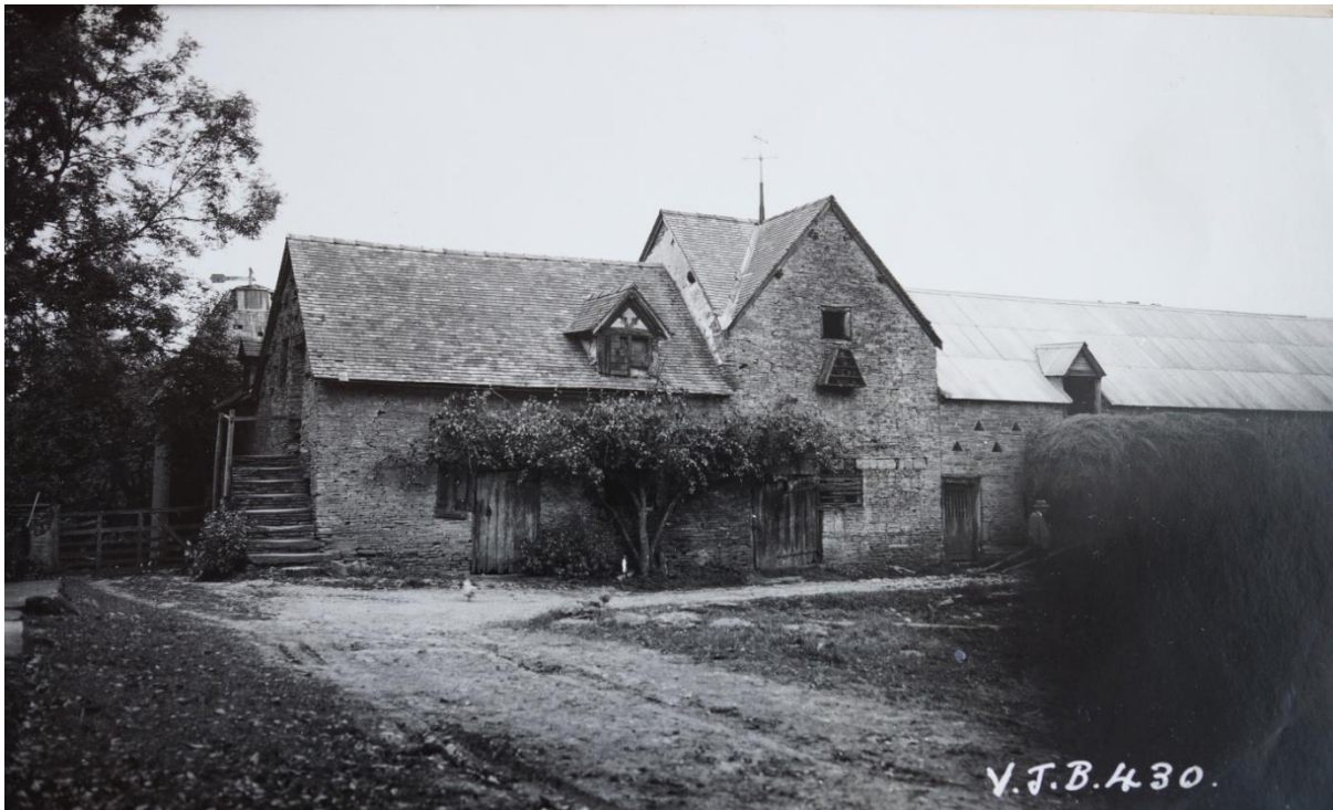
Figure 7. Photograph taken by the RCHME surveyors - survey made in 1933. Note the hop kiln cone visible on the left. Note too the clay tiles on the granary and dovecote roofs, and the corrugated iron roof over the cowhouse and barn. (By kind permission of English Heritage ©)
