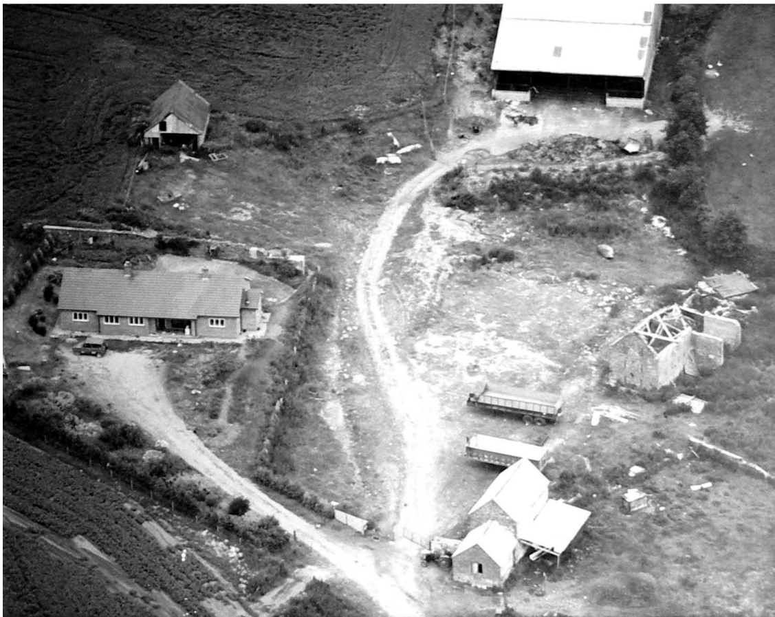
Figure 2. Aerial photo of Carwendy in the mid-1980s showing the bungalow on the site of the old house. The roofless threshing barn lies to the right of the figure 10 on the tithe map
