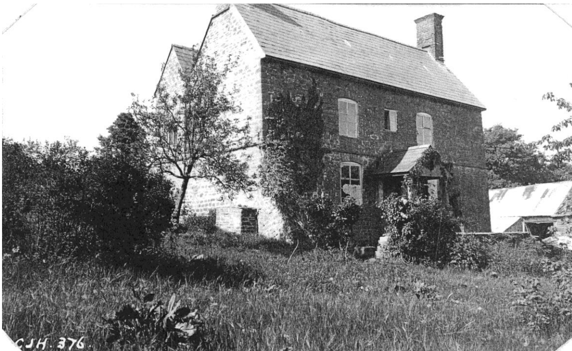
Figure 5. The RCHME photo of the south-east front. Note the threshing barn in the background. ©English Heritage by kind permission
