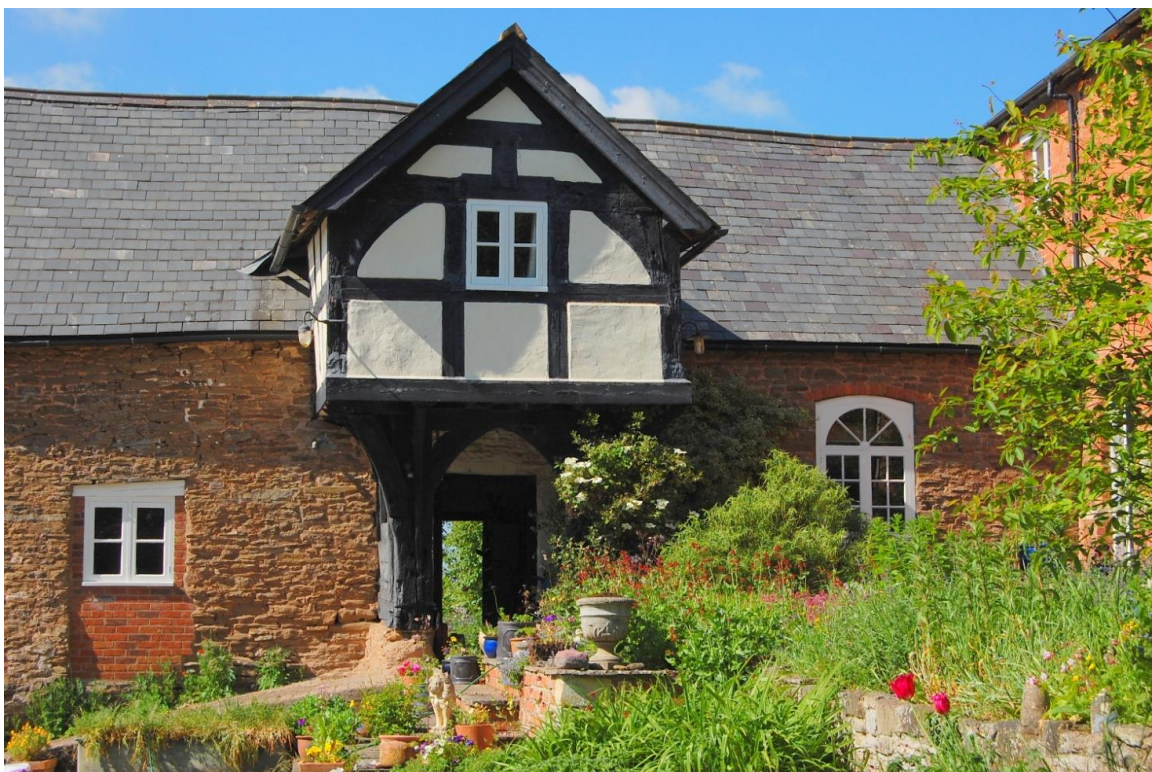
Figure 6. Lower Marston - late 14th-century porch
