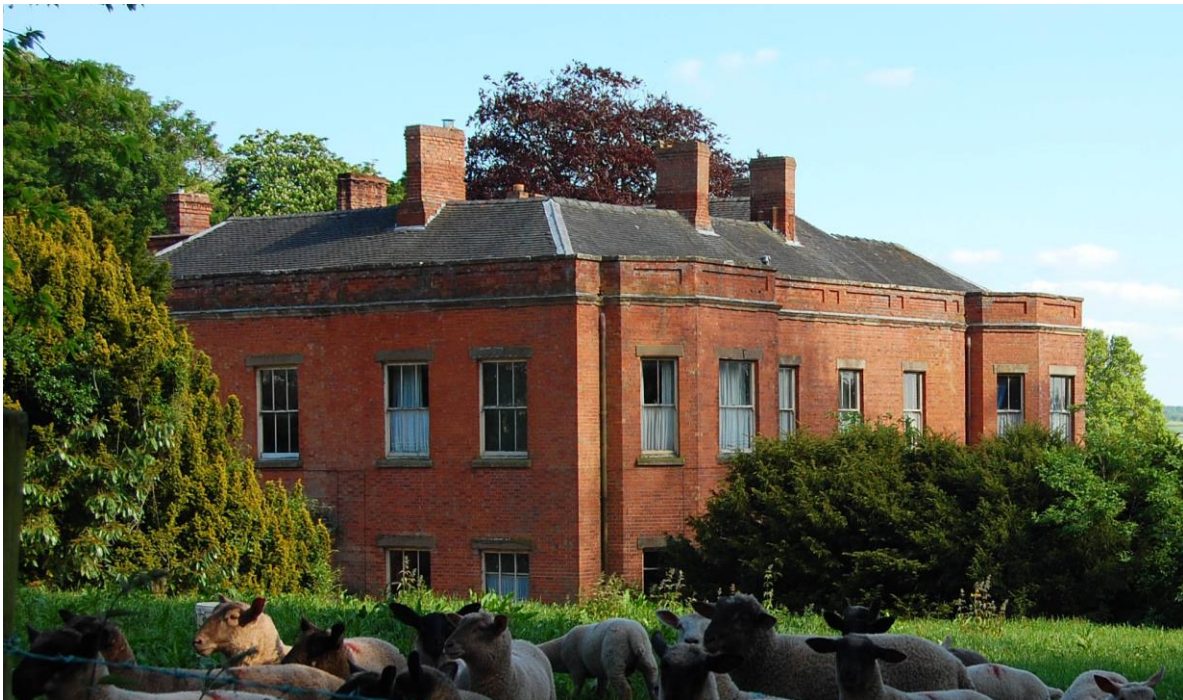
Figure 12. The bow-windowed west front of Buckland House in 2013. The oldest chimney is the second from the left in the picture and is shown in more detail overleaf.
