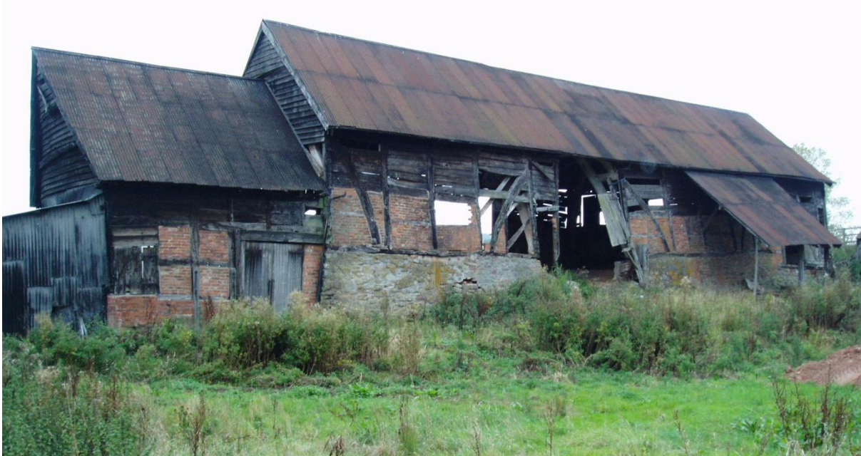
Figure 1. The south-east face of Aylton barn before restoration
