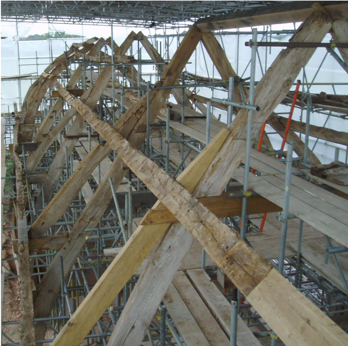
Figure 7. Looking along the exposed crucks
