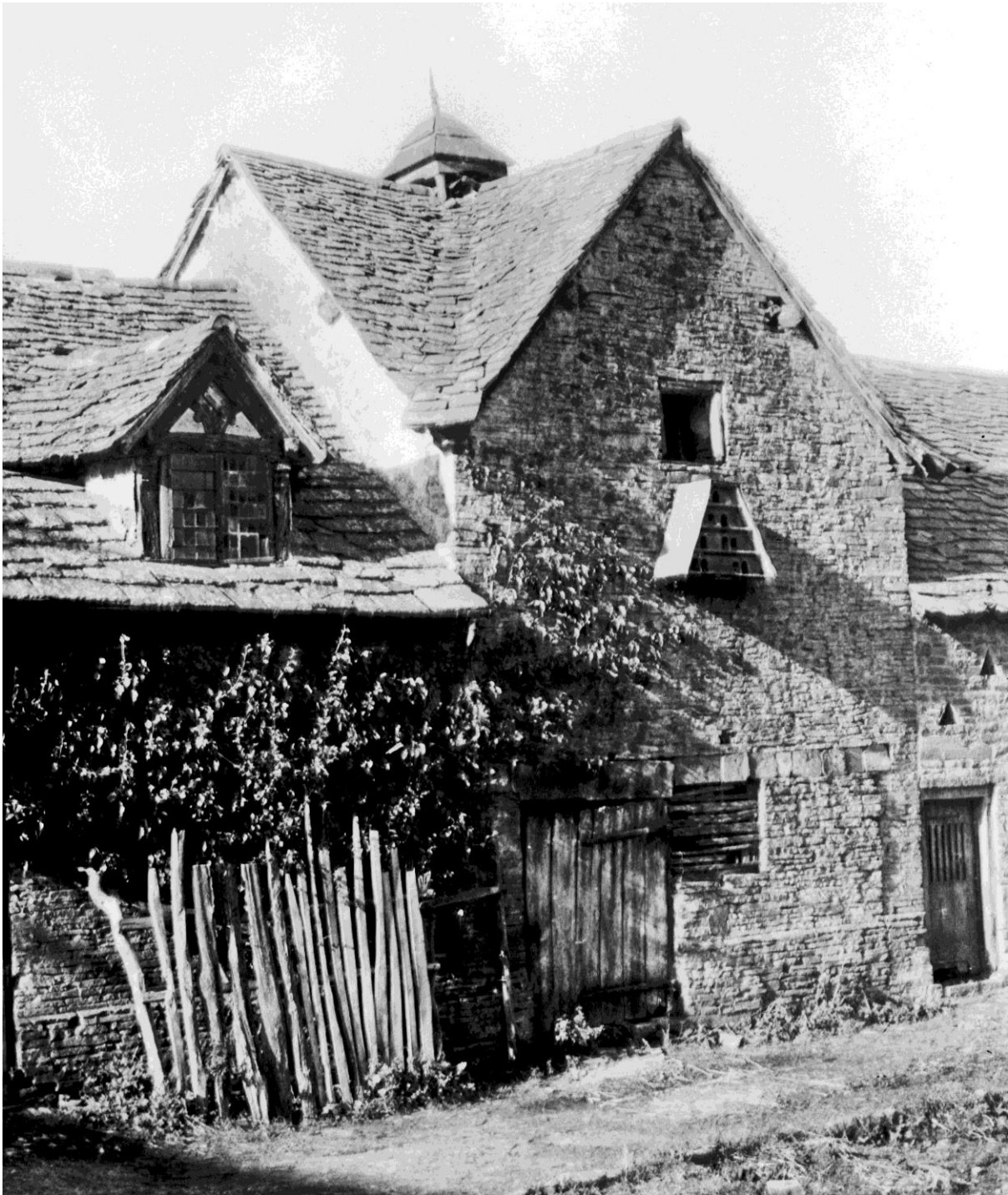
Figure 11. Photograph of the south-east face of the main range, showing to stone tiles on all buildings, the dormer in the 'granary' and the dovecote. Note the gully arrangement of the four-gabled dovecote roof, the box cote below the window and what looks like a louver for the birds to enter on the top. This latter had gone by 1933 after the re-roofing had taken place (see Fig. 7).
