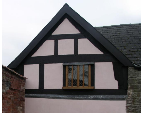
Figure 16. Re-made orielle window in 2015
