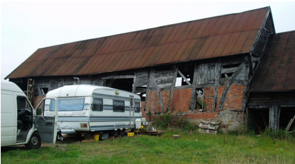
Figure 2. The back of the barn before restoration
