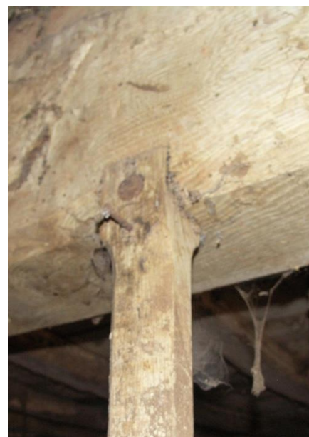
Figure 18. Chamfered and pegged beams and uprights of stalls.
