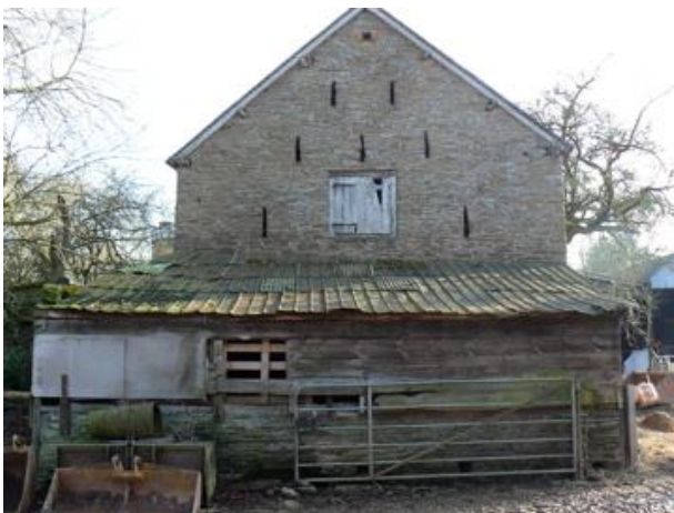
Figure 22. Gable of barn to north-east of farmyard.
