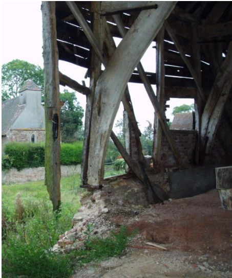
Figure 2. A cruck on the south-east face with the church in the background
