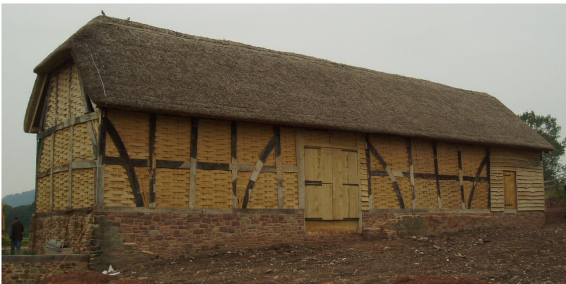
Figure 8. The finished barn with repaired timbers
