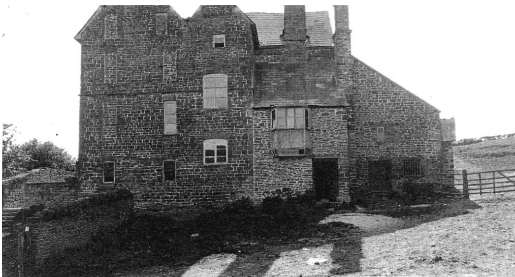
Figure 4. The RCHME photograph of the north-eastern front of Carwendy, which faces the threshing barn and is the bottom face of the house in the plan above. The truncation of the chimneys is in the original photograph. No notes were made on item 6, 'Grounds'. ©English Heritage by kind permission
