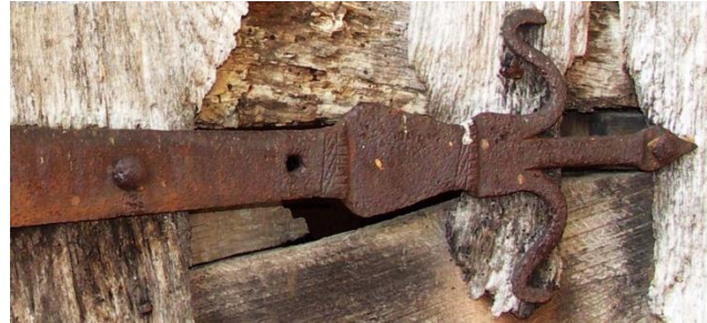
Figure 21. One of pair of strap hinges on barn door
