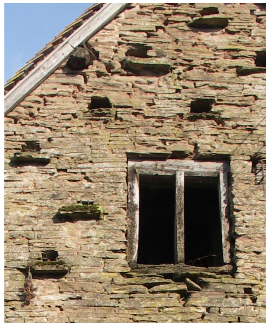
Figure 10. Detail of the inbuilt gable-cotes.
