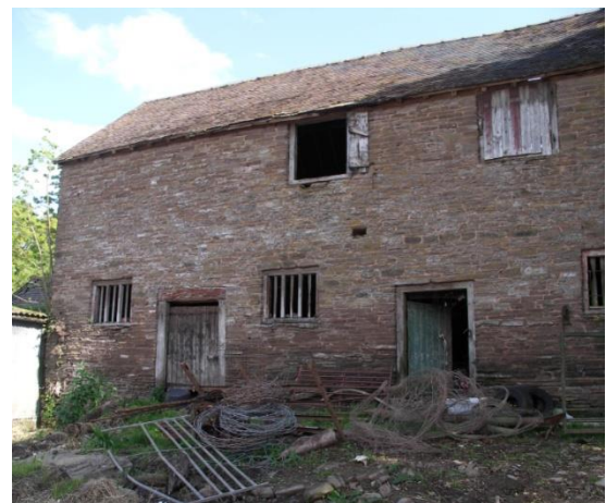
Figure 23. Building to east side of farmyard.
