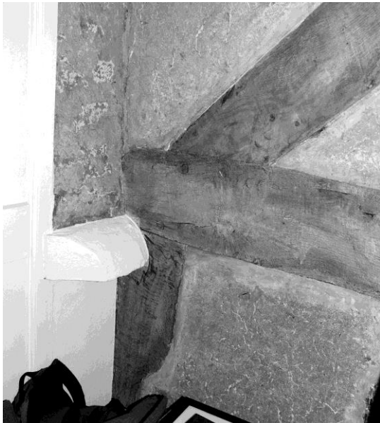
Figure 19. Junction of the older kitchen block roof (to the right) and a timber of the sitting room block (RS)
