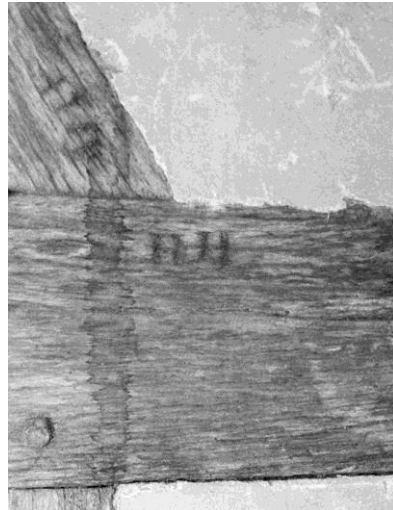
Figure 24. Punched carpenters' marks (RS)
