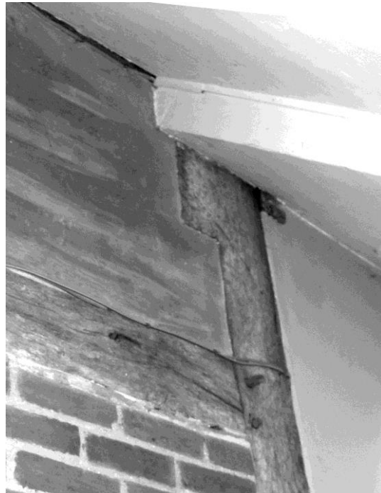
Figure 20. Possible attachment trench for a pentice support (RL)
