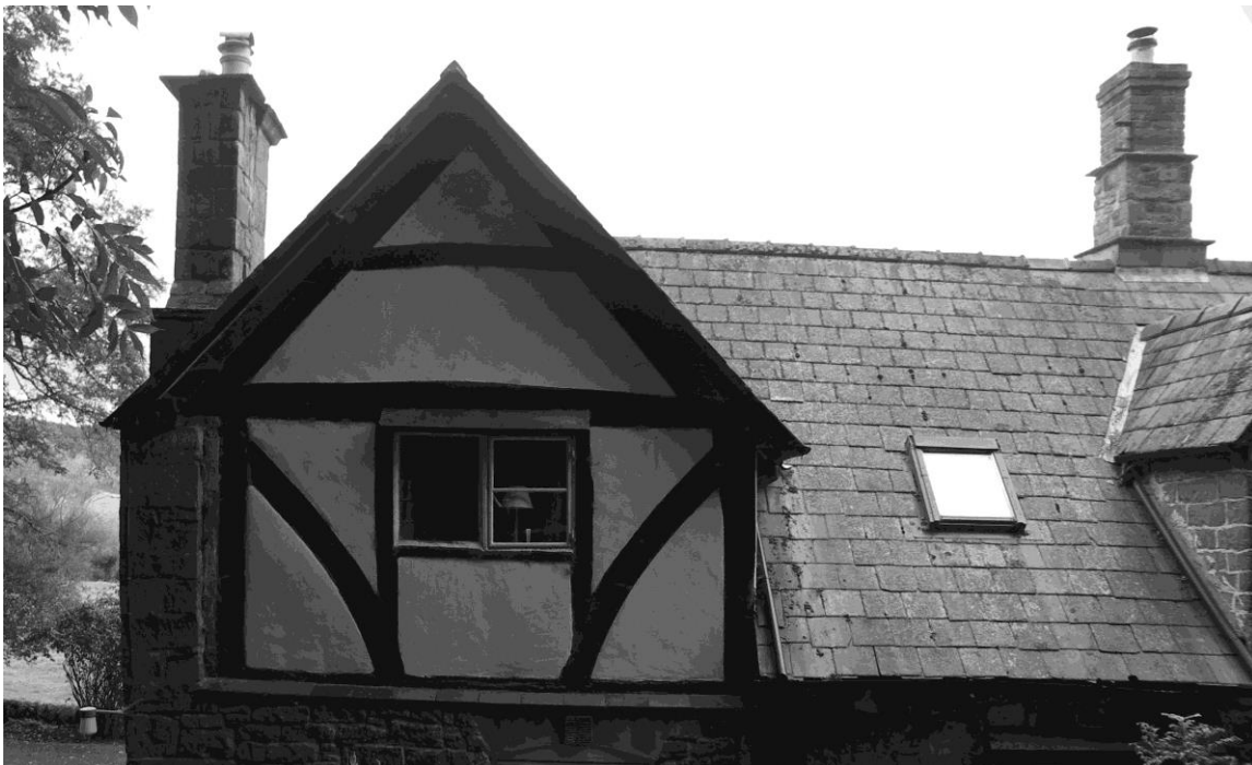
Figure 3. Exposed timber-framing at rear of farmhouse
