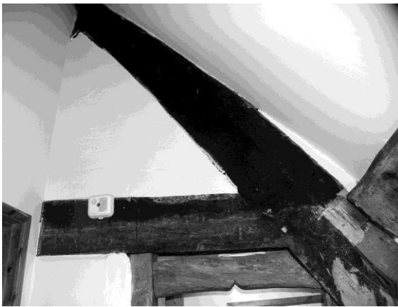
Figure 13. Cruck in inserted upstairs passage. the door head is modern The re-used timber in the E gable-end (not visible outside) may have come from an earlier building.
