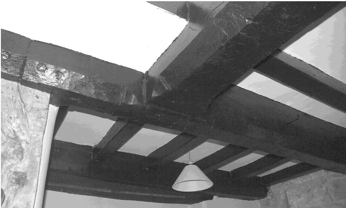
Figure 5. Inserted ceiling in S cross-wing of farmhouse
