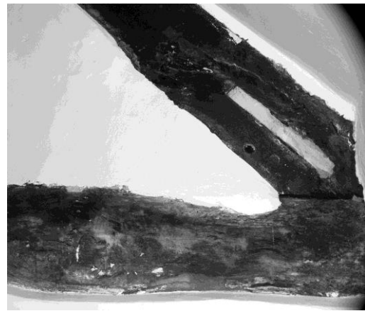
Figure 13. Cruck in inserted upstairs passage. the door head is modern The re-used timber in the E gable-end (not visible outside) may have come from an earlier building.
