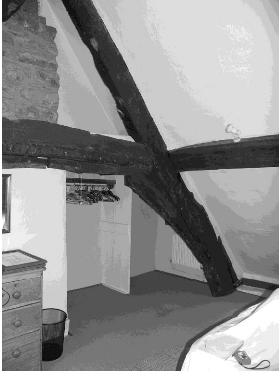
Figure 7 Open cruck in first-storey bedroom in farmhouse, E wall.
