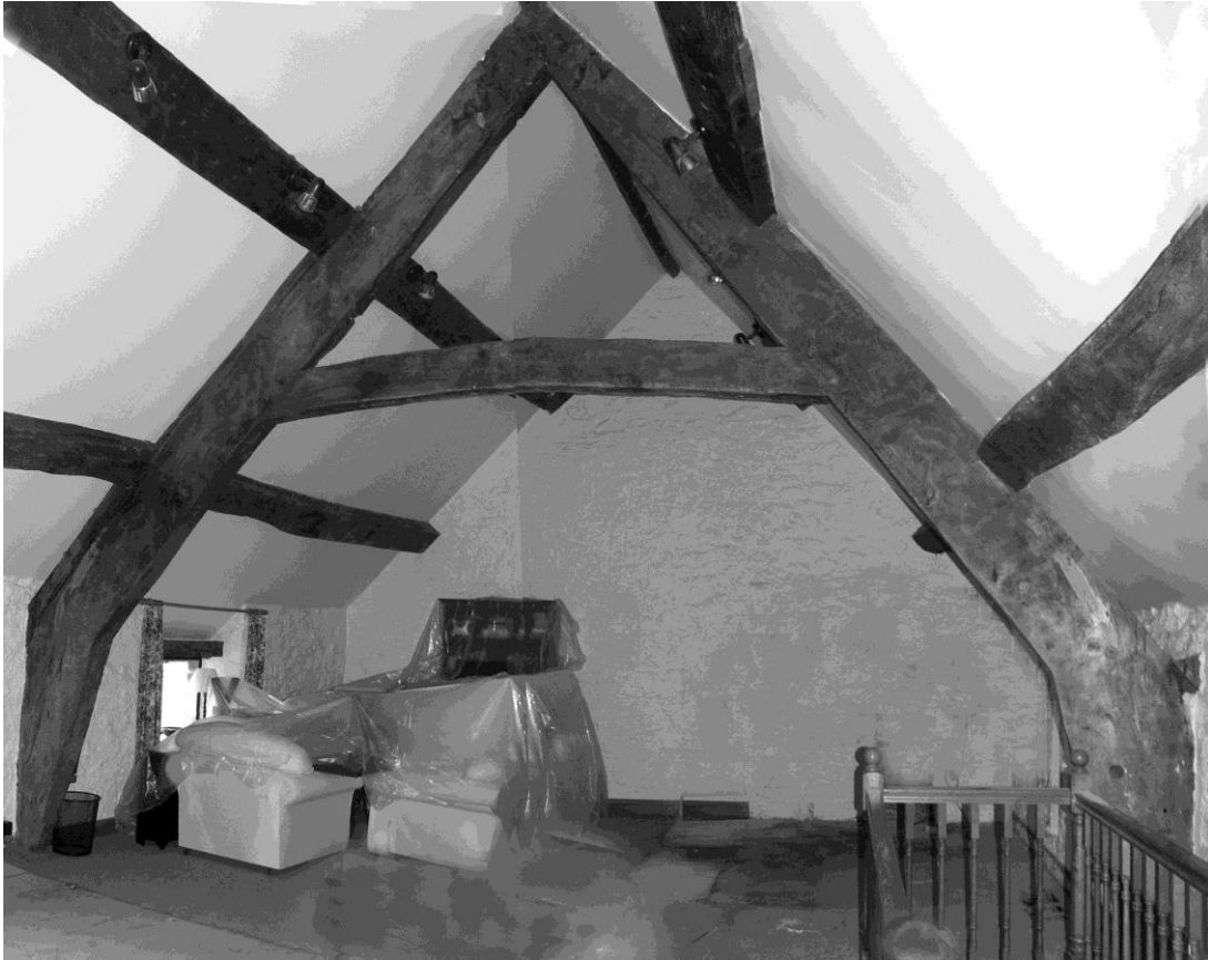
Figure 23. The beams in the malthouse. Two photographs were merged because of the difficulties of including both crucks in one shot.
