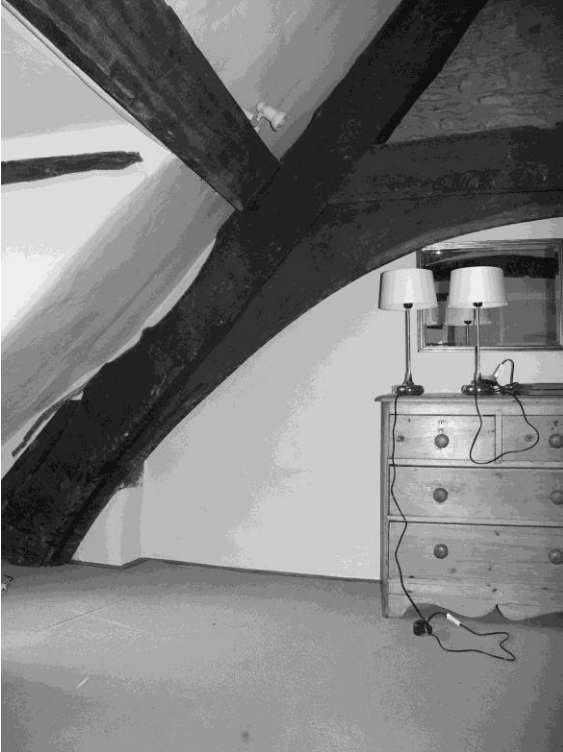
Figure 6. Open cruck in first-storey bedroom in farmhouse, W wall.
