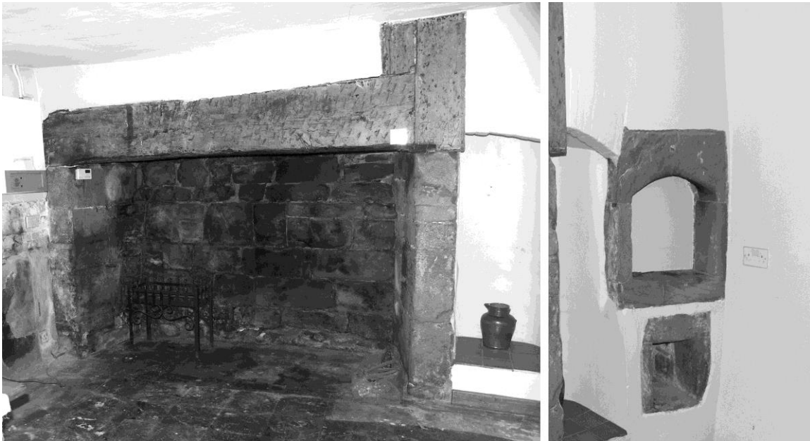
Figure 16. Kitchen fireplace and to the right the apertures for the bread oven and fire.
