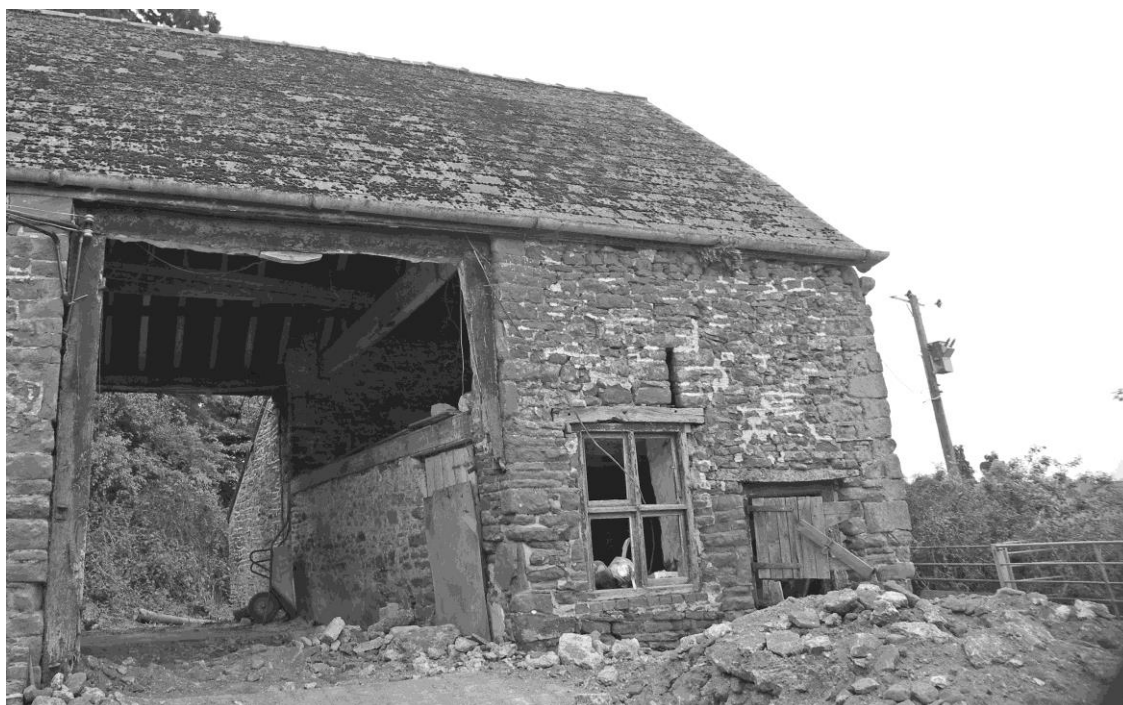
Figure 5. North-eastern side of the threshing barn
