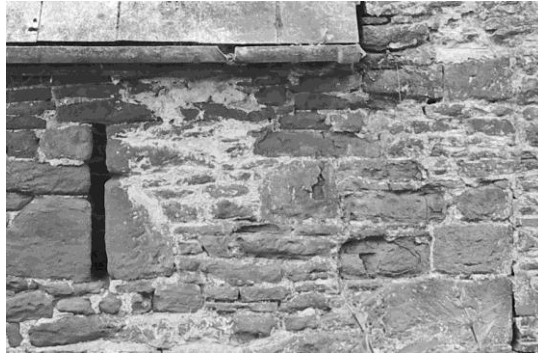
Figure 8. Rear of threshing barn showing junction with building nearer the house
