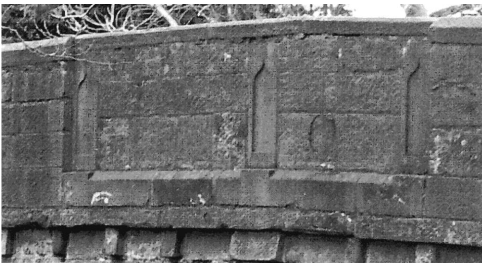
Figure 2. Old Forge Bridge - details of the parapet
