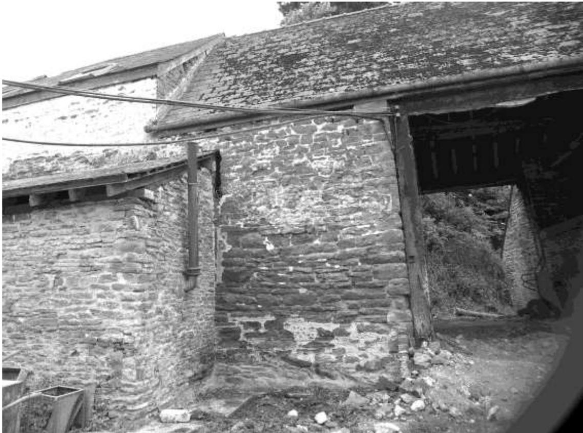
Figure 6. North-eastern side of the threshing barn, at its junction with the newer part next to the house. This gives a fair indication of the various buildings which have been added to the original barn
