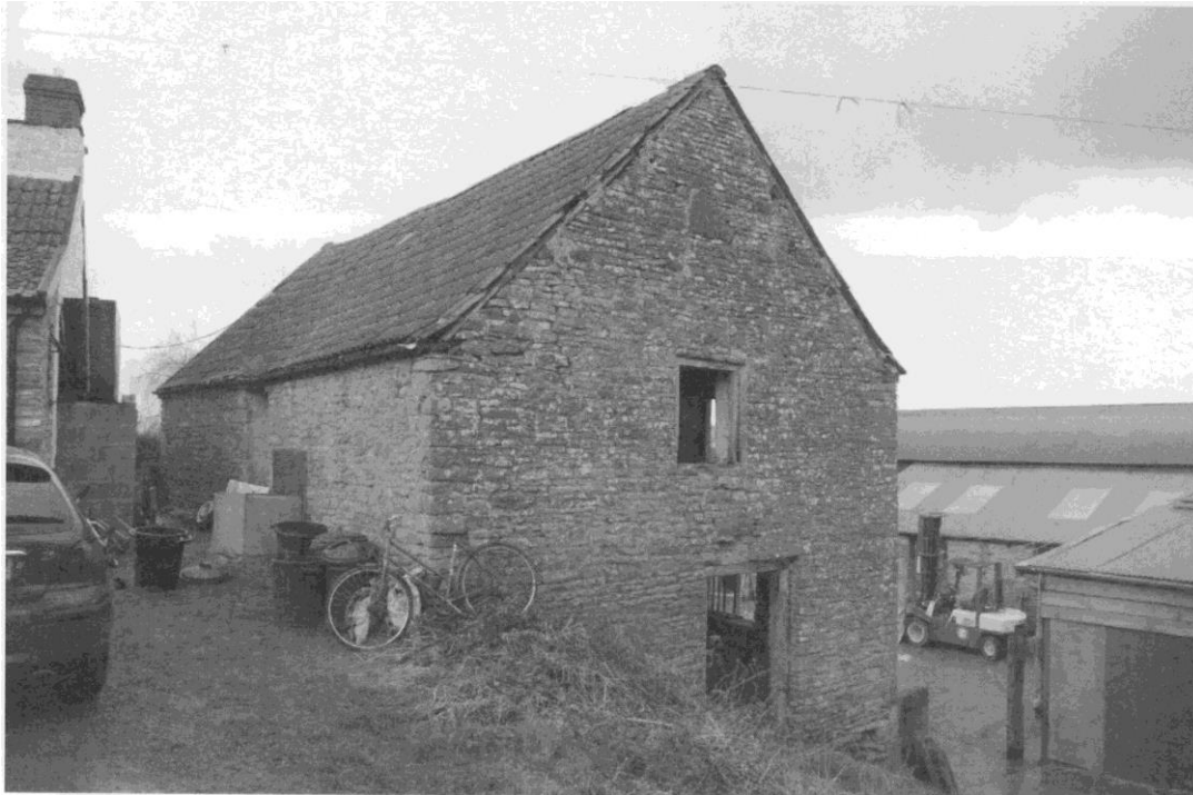
Figure 8: The south and east elevations, showing how the building terraces into the hill slope
