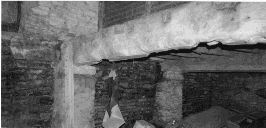
Figure 13: Bridging beam and additional reinforced pillars
