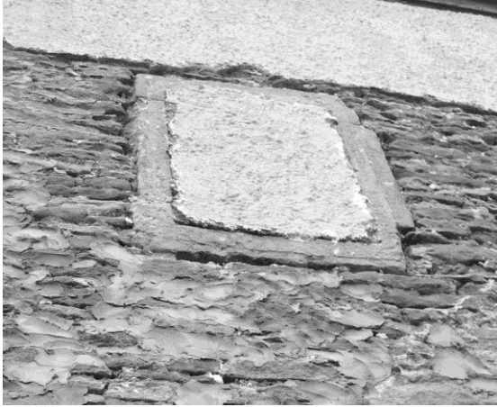
Figure 6: Stone window frame on east face
