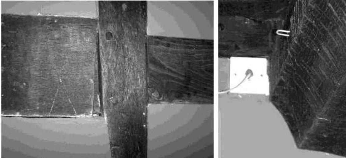
Figure 9 carpenter's mark on W wall of central block, and chamfer on E-W beam, both downstairs
