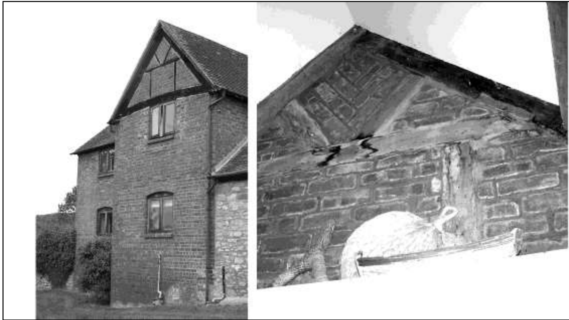
Figure 17 W wall of building 8
