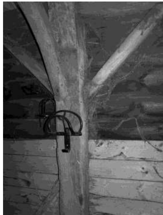
Figure 13 Reused timbers in Newton's outbuilding
