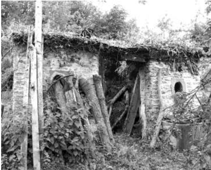
Figure 22 E wall of building
