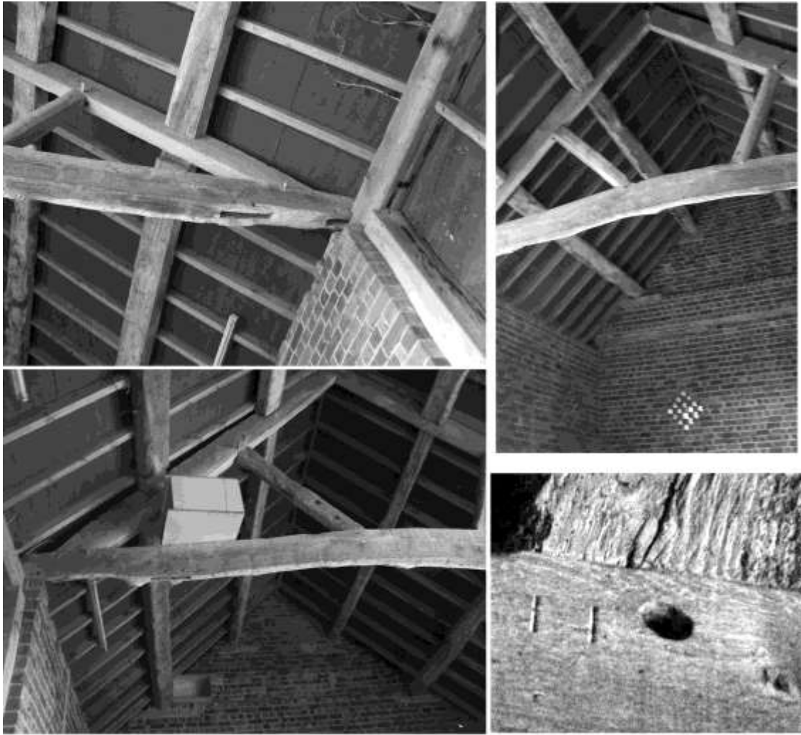
Figure 19 Building 10 roof timbers
