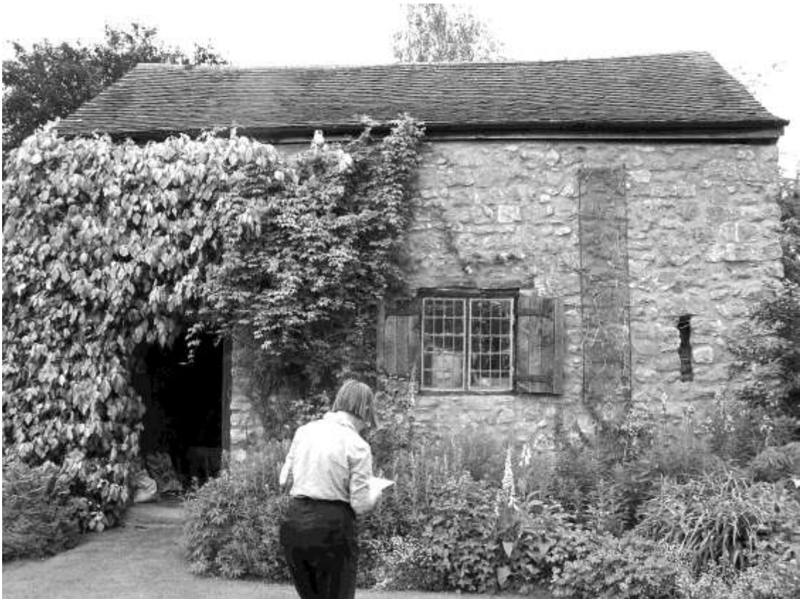
Figure 15 W facade of building 6a
