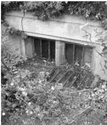
Figure 17 Exterior cellar window
