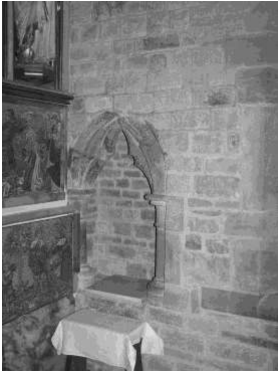
Figure 3 Piscine found in walls
