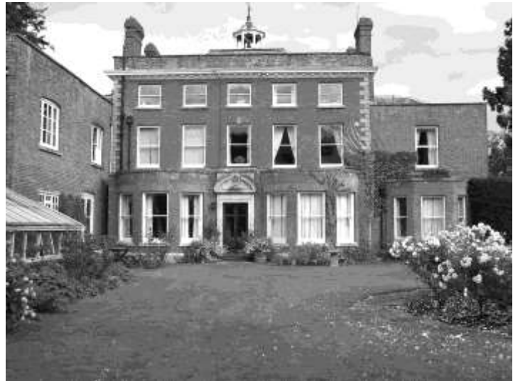
Figure 20 Rear of the Court
