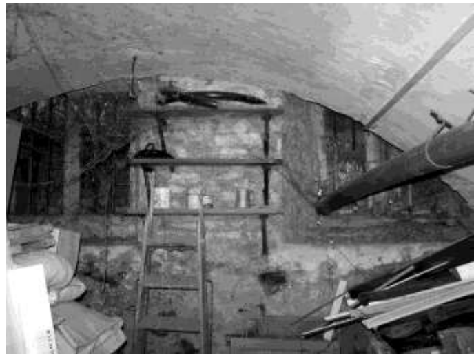
Figure 18 Internal cellar windows
