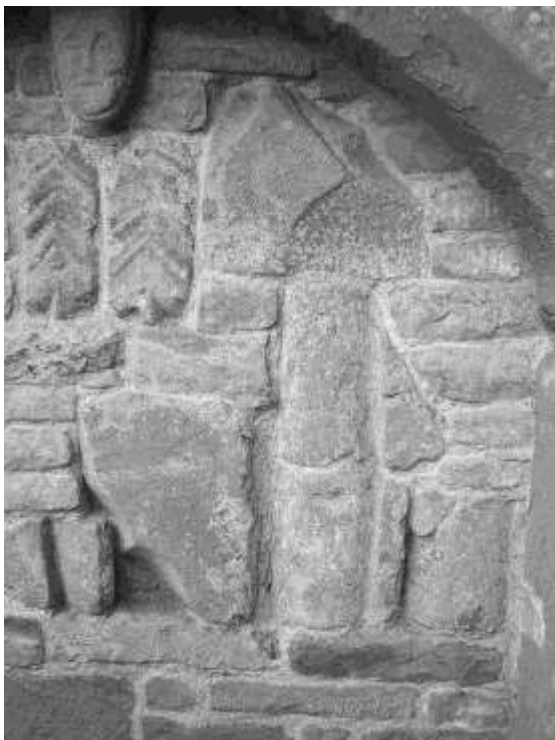
Figure 5 Outside of N Doorway
