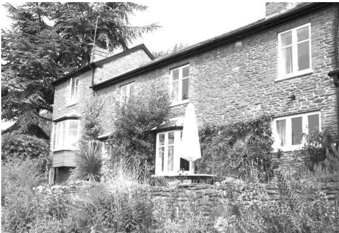
Figure 15 Old Grove House - SW side overlooking stream
