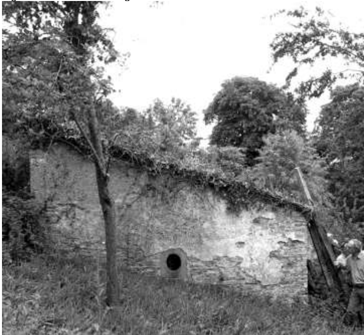
Figure 23 S wall of building
