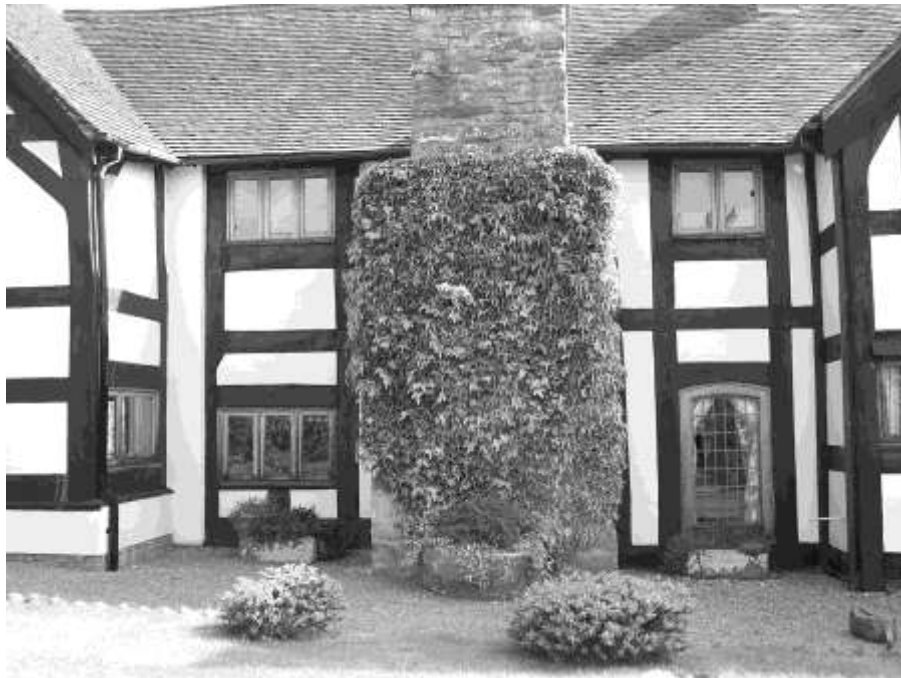
Figure 4 N facade with pentice and porch removed
