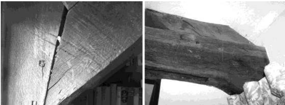
Figure 10 carpenter's marks at E end of central block
