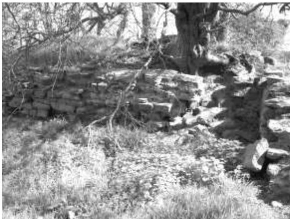
Figure 11 walls of 'mill' viewed from NW
