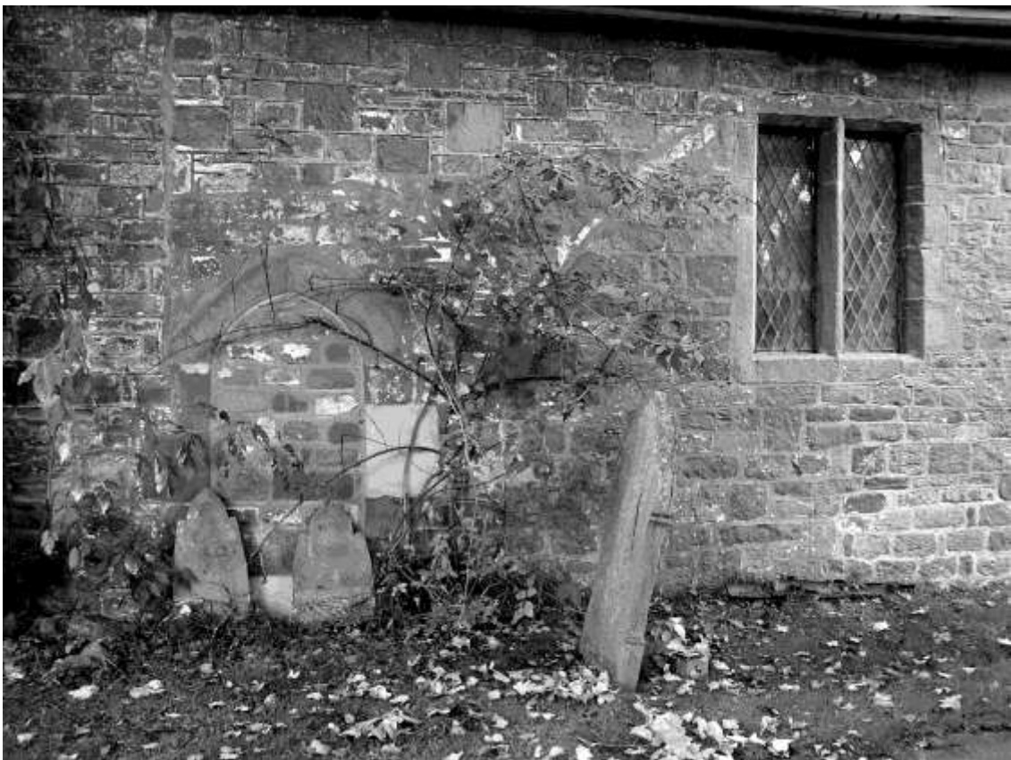
Figure 3 S wall of the nave
