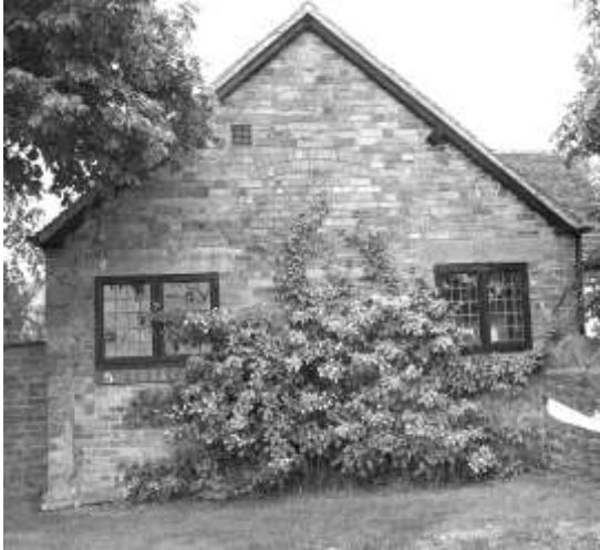
Figure 15 Building 2 from W
