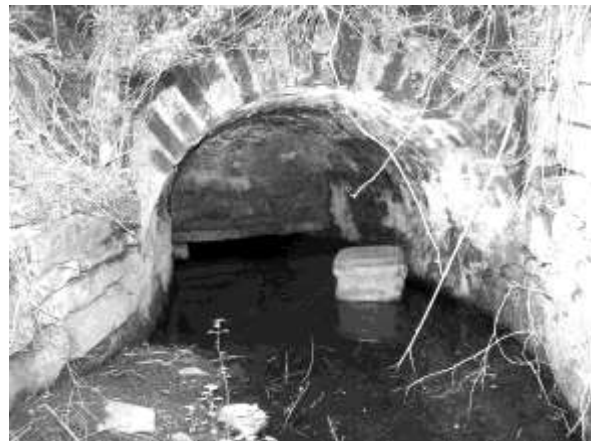
Figure 12 culvert looking NW
