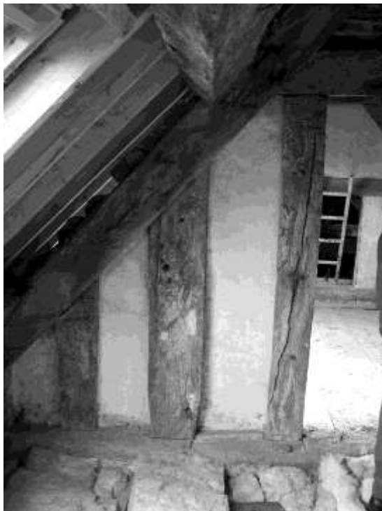
Figure 8 Timber framing in house loft
