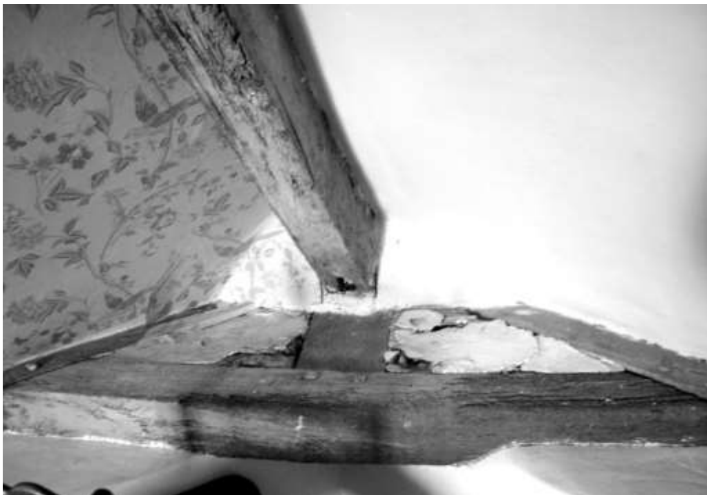
Figure 16 Corner of NE block showing roof timbers
