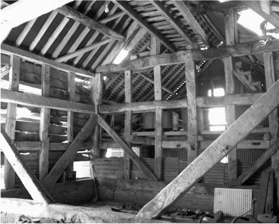
Figure 5 Building 8a showing re-used timbers
