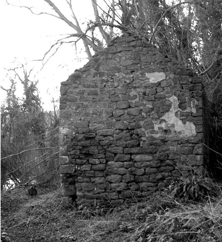
Figure 4 End wall of 653 showing blocked up doorway on left (R Lowe)
