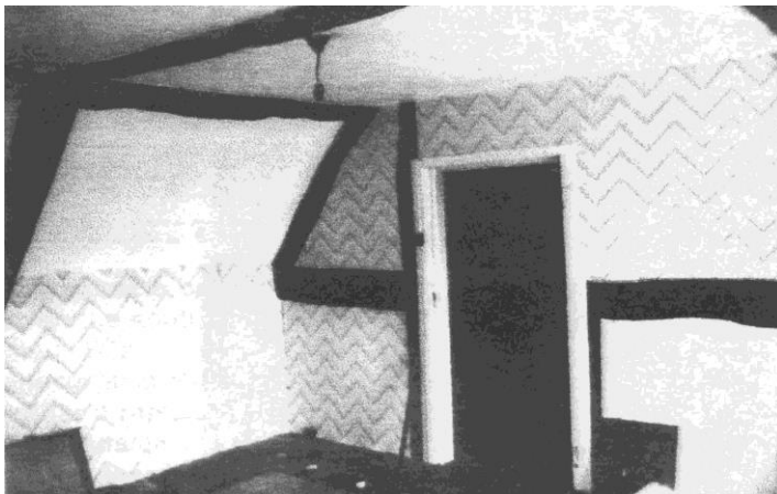
Figure 4 3rd storey loft with possible re-used timber (G Wells)
