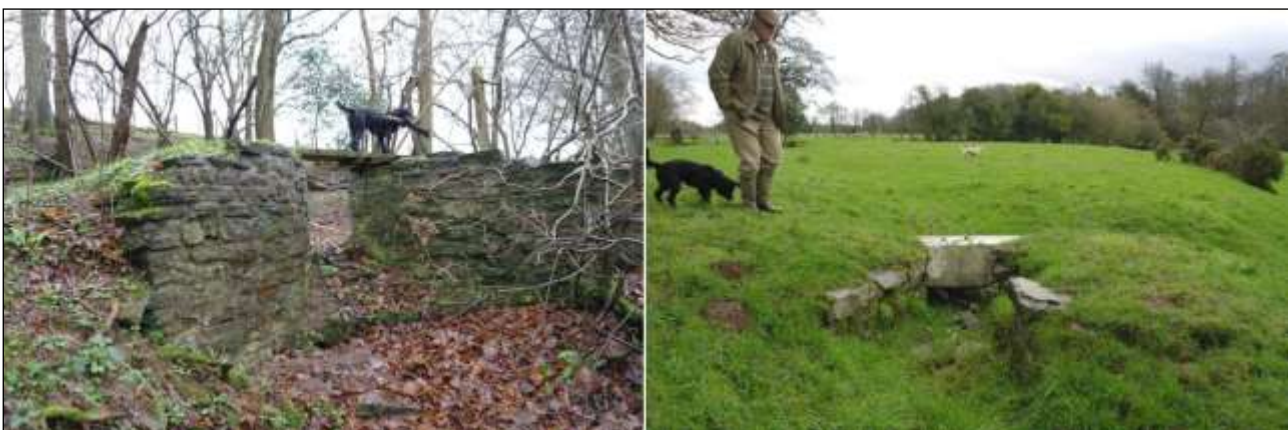
Left: Stone discharge sluice in the main southern channel as it skirts the wooded northern slopes along the contours feeding the water meadows on the south side of the Arrow below and down stream from Grove Farm.
